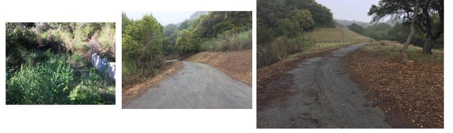
After the work had been completed, the road is extensive, serves as a fire break, and allows access to key drainages mid-slope below the Bayview Fire Road. Approximately 2,500 feet of roadway was uncovered extending past Loch Haven Ct. and 150 cubic yards of vegetation was removed in the process. The SRFD will be able to use this road in the future to help suppress any wildfire threat to the community. This road is now accessible for emergency vehicles and pedestrians.
