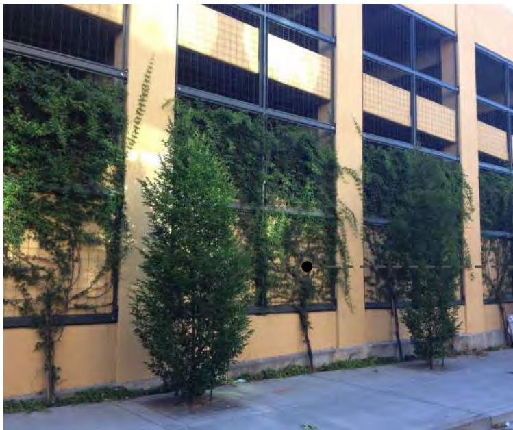
GROUND FLOOR OPENING TREATMENT
