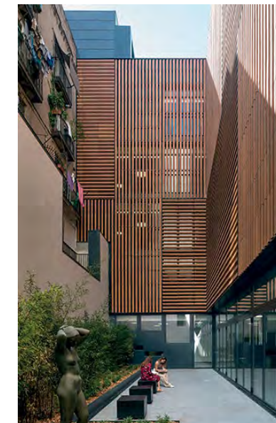
SHADING SKIN ON EAST & WEST FACADES
