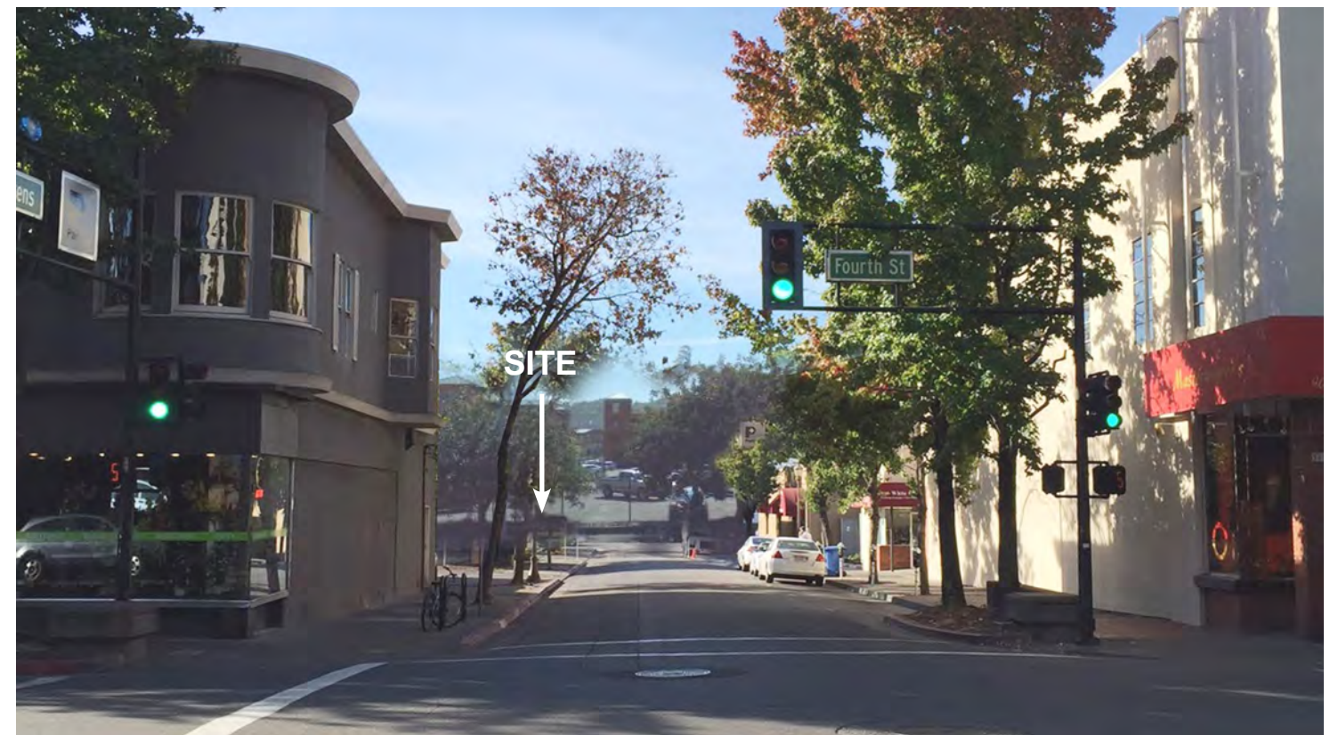
View from Lootens Place (looking south)
