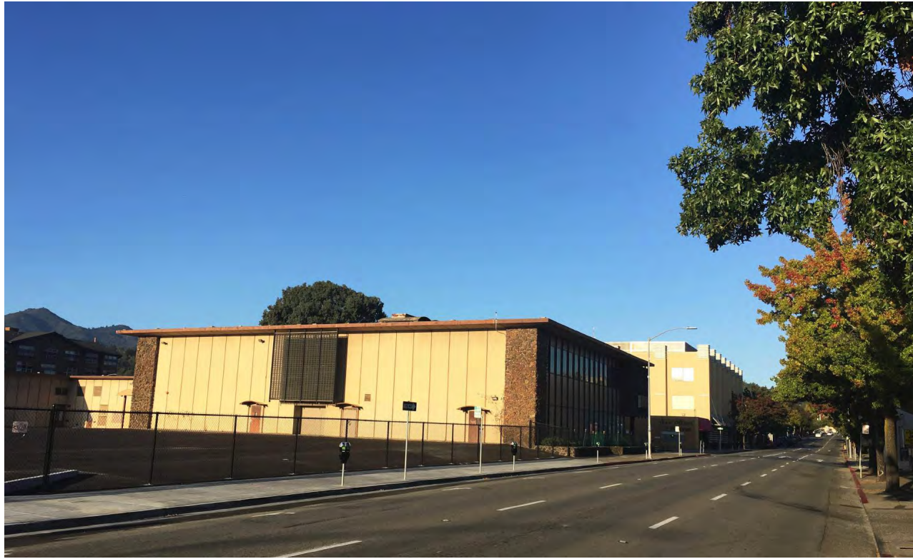
1 VIEW FROM 3RD ST
