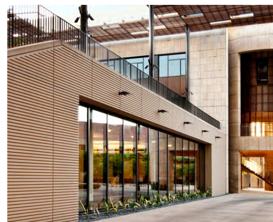
ENTRY & BASE OF BUILDING
