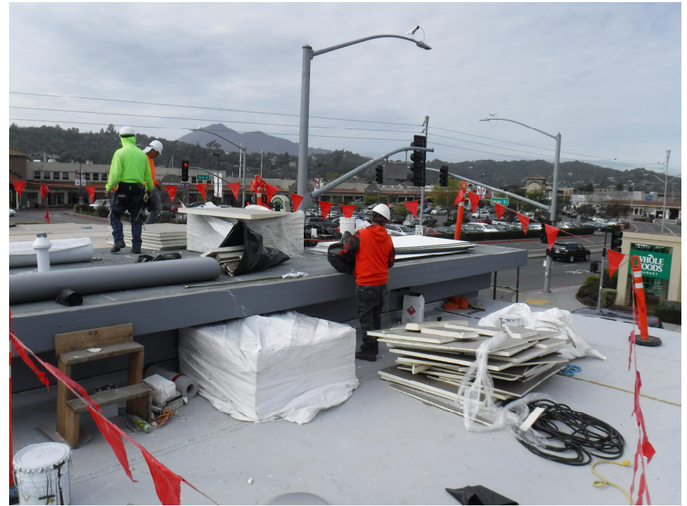
February progress picture – Training Classroom TPO Roof Installation
