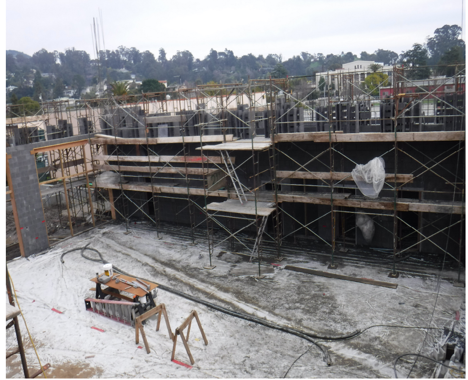
January progress pictures – Fire Station CMU Installation and Scaffolding
