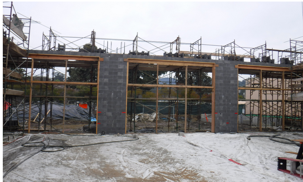
January progress pictures – CMU and Door Framing for Bay Room
