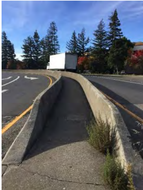
Sidewalk from Lucas Valley Road to Southbound US 101 Transit Stop
