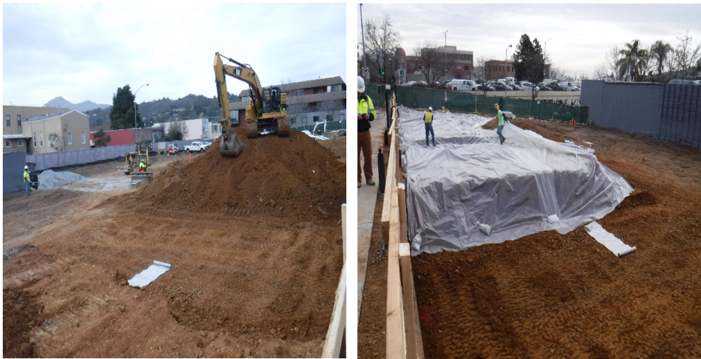
February progress pictures – Over excavation of site and protecting area from rain.
