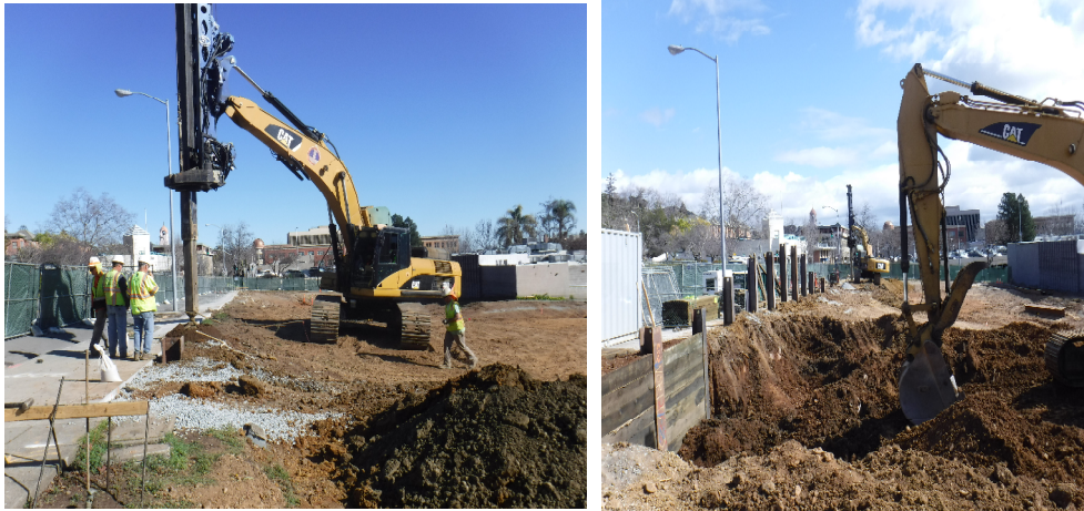
February progress picture – installation of the shoring beams and
