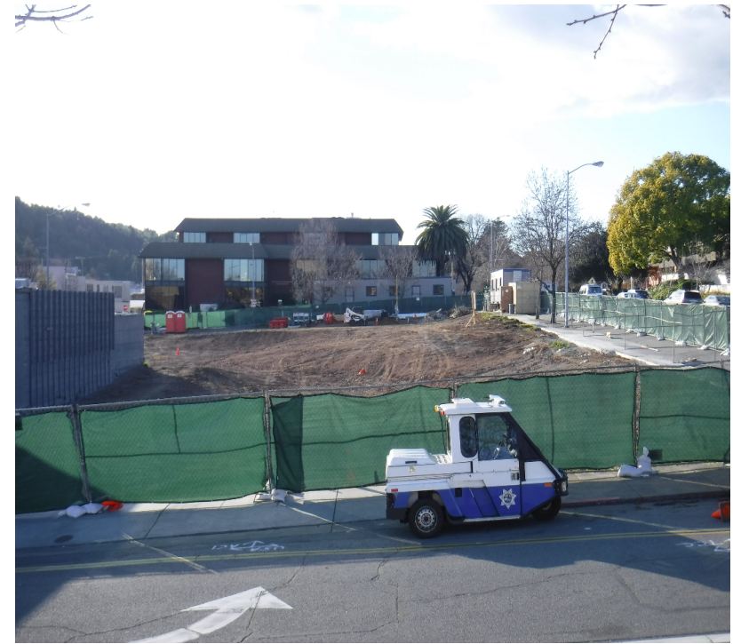
February progress picture – Overview of project site
