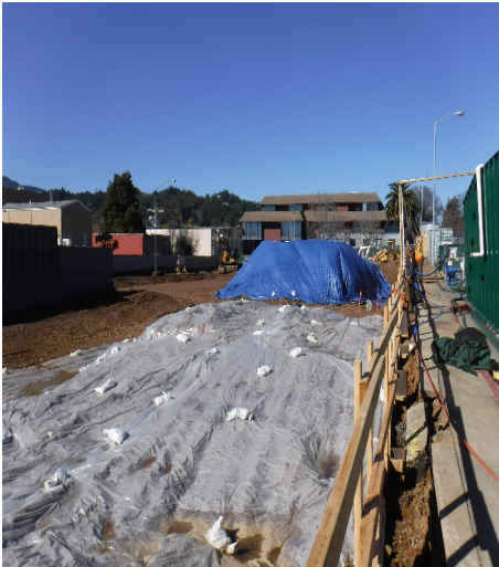
March progress picture – installation of the baker tanks and covering of the stockpiles
