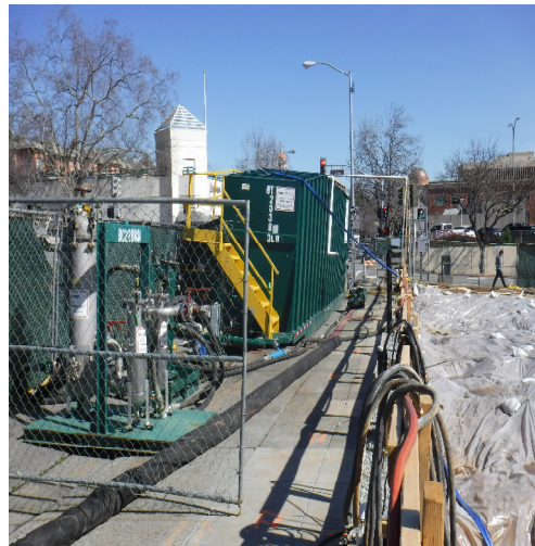
March progress picture – installation of the baker tanks and covering of the stockpiles
