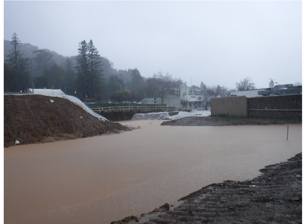
March progress picture – Overview of project site during a rainy day
