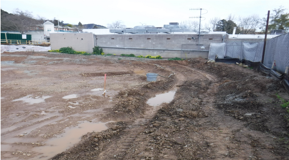
March progress pictures – pumping system of the site.
