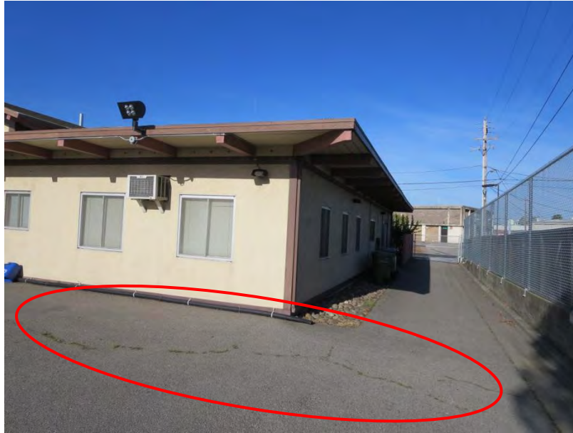
Photo 5: Station 54, Possible Soil Consolidation
