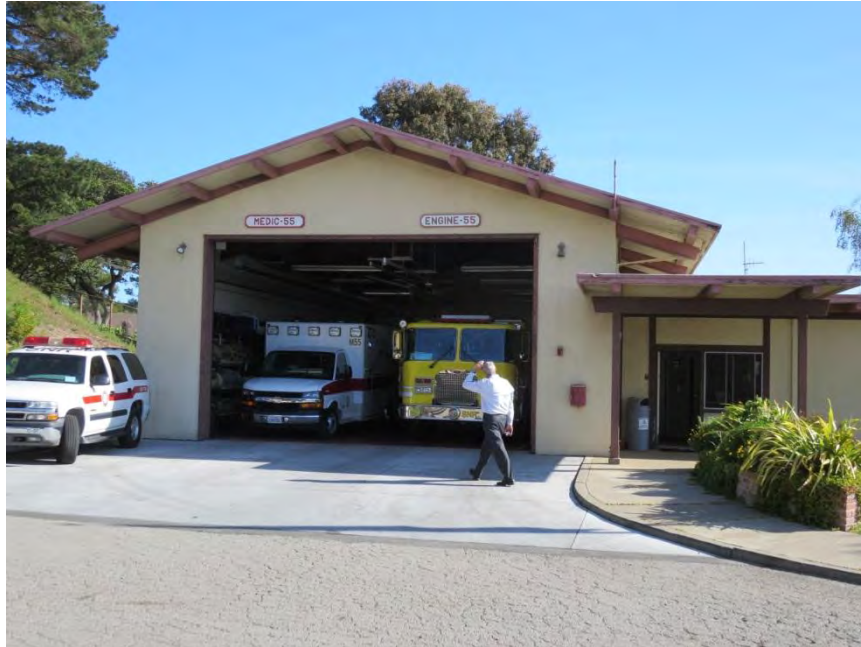
Photo 6: Station 55, Exterior of the Building
