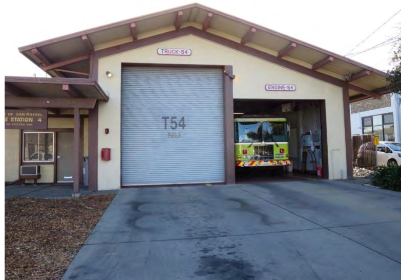
Photo 1: Station 54, Exterior of the Building
