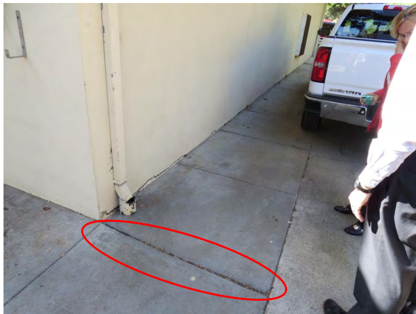
Photo 11: Station 55, Possible Soil Consolidation
