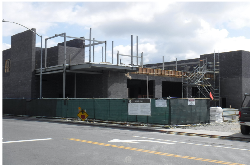
April progress picture – Looking Northeast to Fire Station Building
