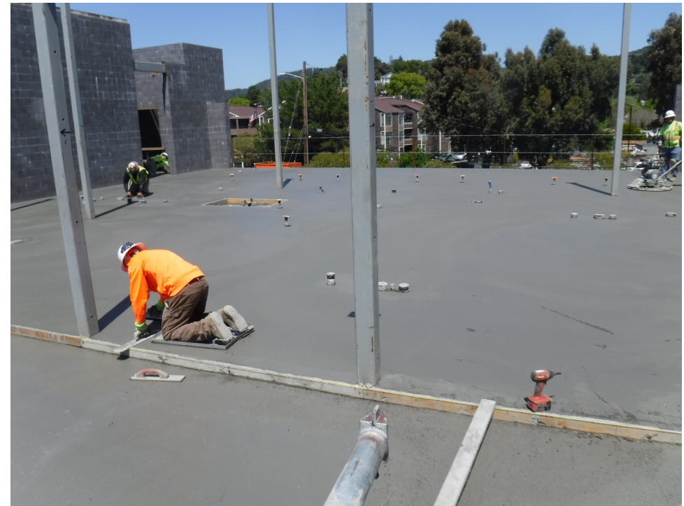
April progress picture – Fire Station 2 nd Floor Elevated Slab. Concrete Finishing.
