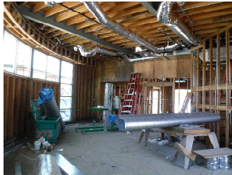
April progress pictures – (left) Classroom Lath and Flashing; (right) Classroom Ductwork
