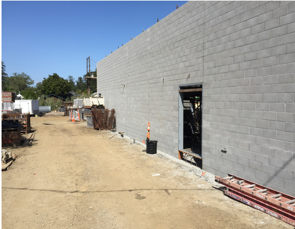
April progress pictures for Fire Station 57
