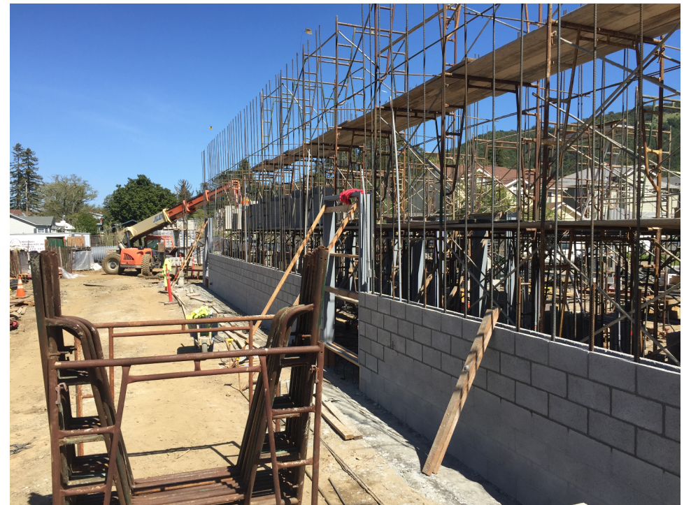
April progress pictures for Fire Station 57
