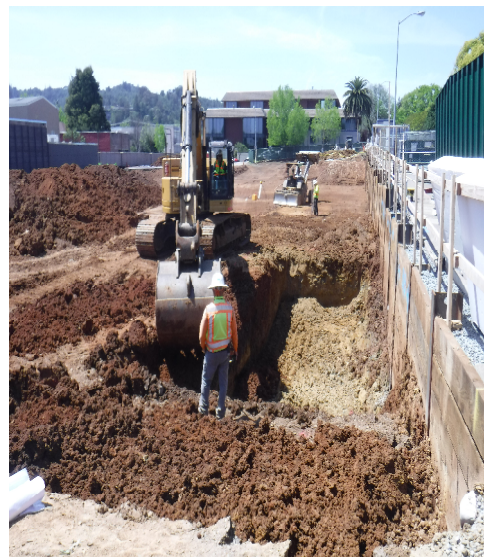
April progress picture – over-excavation of the contaminated material and unsuitable areas
