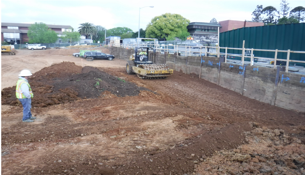
April progress pictures – using wheel for compaction of over excavated areas
