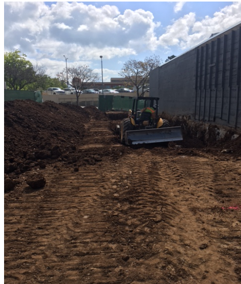
April progress picture – over-excavation of the contaminated material and unsuitable areas
