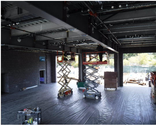
May 2018 progress pictures – 1 st Floor Fire Station Apparatus Bay; and Training Classroom
