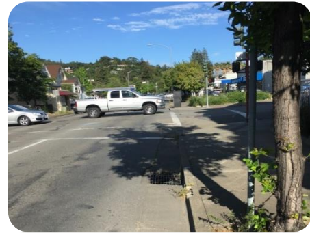
Curb and drainage on 2 nd Street
