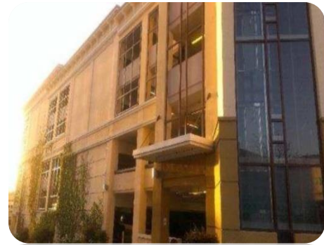
3 rd and C parking structure
