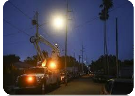
Installation of a new LED street light
