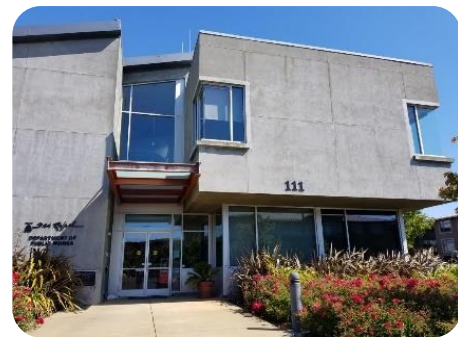
Public Works offices
