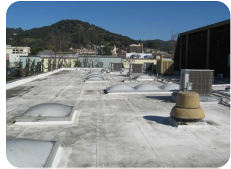
B Street Community Center Roof
