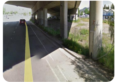
Bellam Blvd under the Highway 101 overpass
