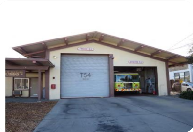
Front of Fire Station 54
