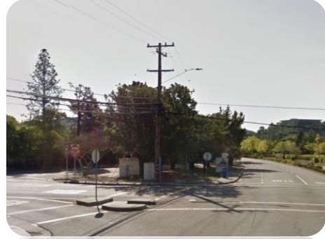
Example of overhead utilities
