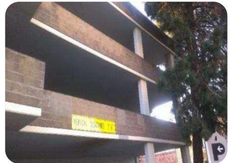
3 rd and A parking structure
