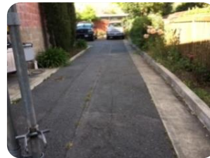
Driveway at Fire Station 56
