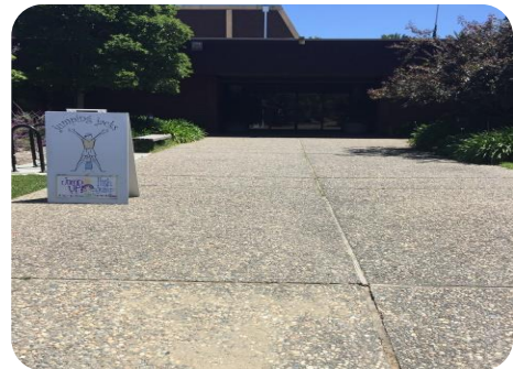
Concrete patio facing front entrance
