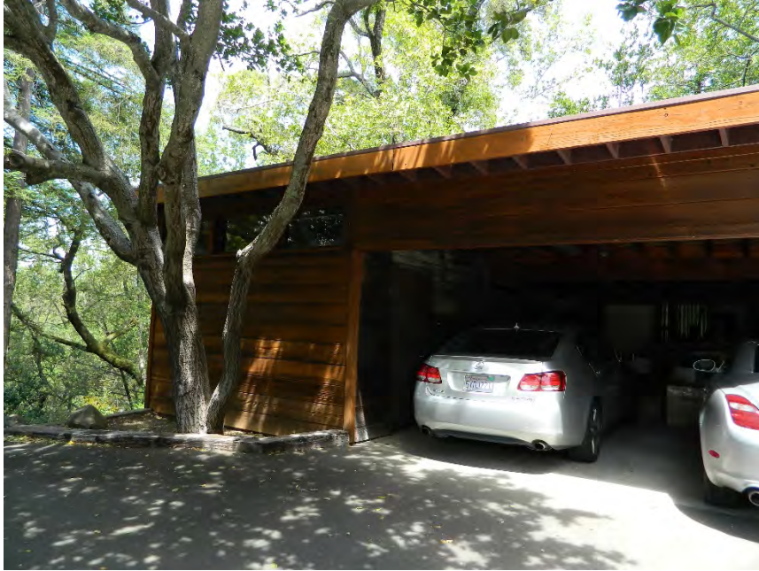
Photo showing the carport, facing north.
