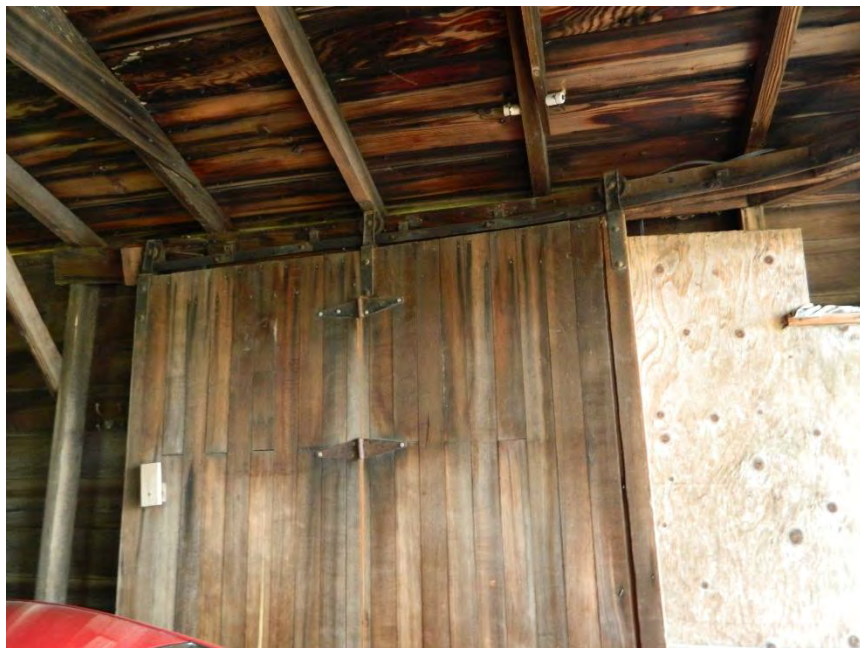
Photo showing the interior of the garage and the original sliding barn-door and track railing.
