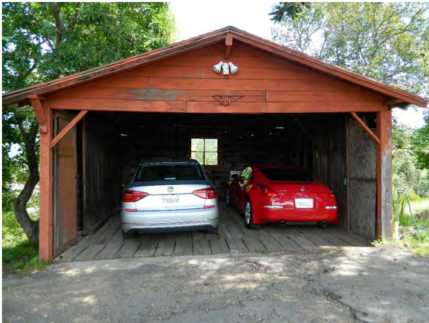
Photo showing the west elevation, facing east.
