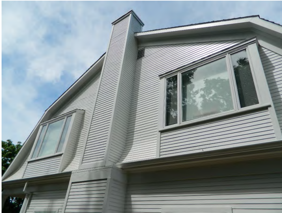
Photo showing the south elevation, facing north/northwest.
