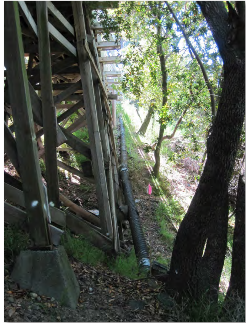
Photo from below bridge, facing south.
