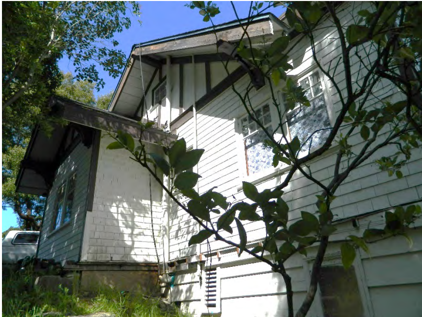
Photo showing the south elevation, facing north/northwest.
