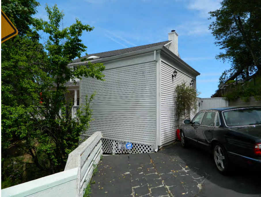
Photo showing accessory building, facing north/northwest.
