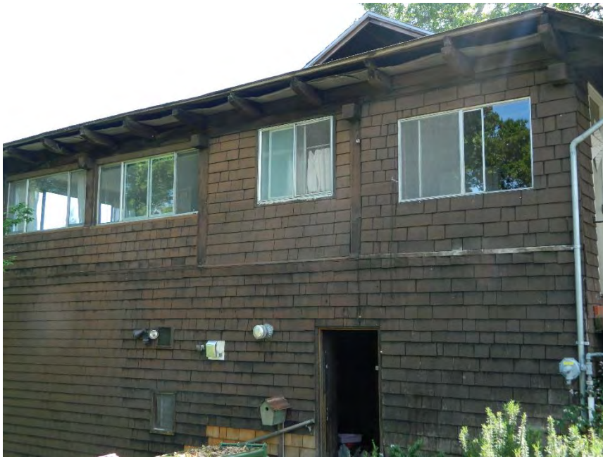
Photo showing the north elevation, facing east/southeast.
