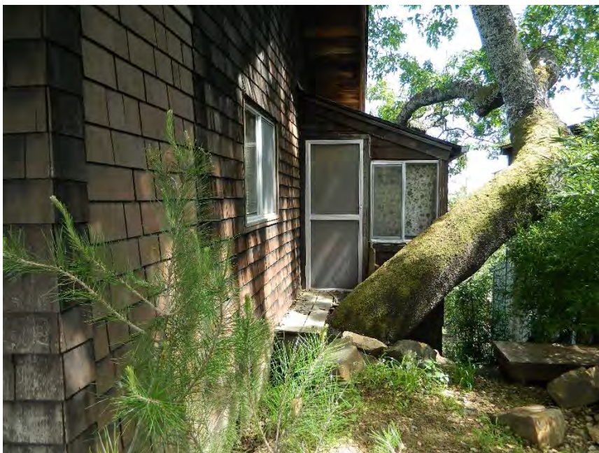
Photo showing the south elevation, facing west.
