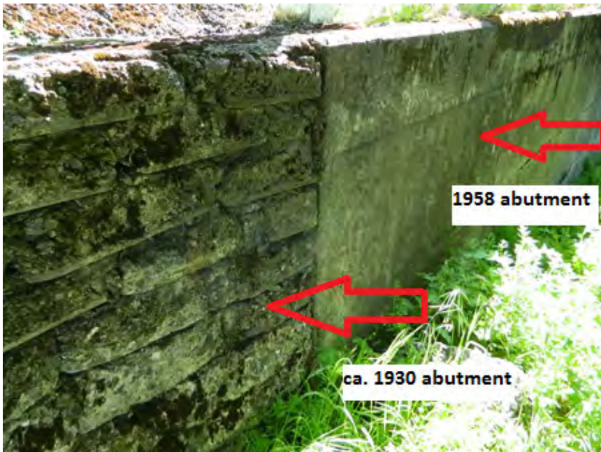
Photo showing ca. 1930 abutment and the 1958 abutment.
