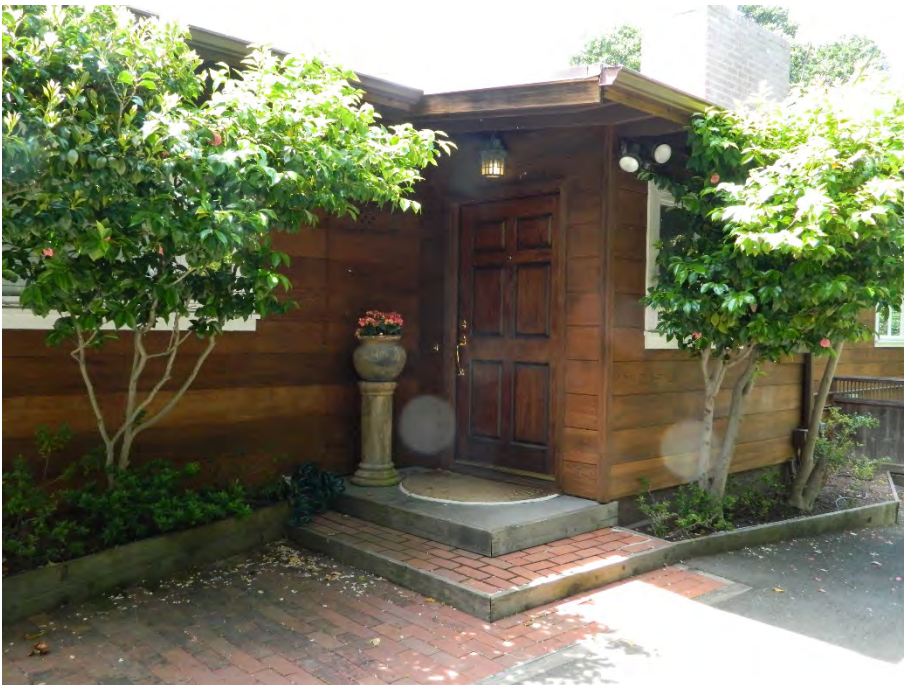
Photo showing the recessed front entry along the northeast elevation, facing southwest.
