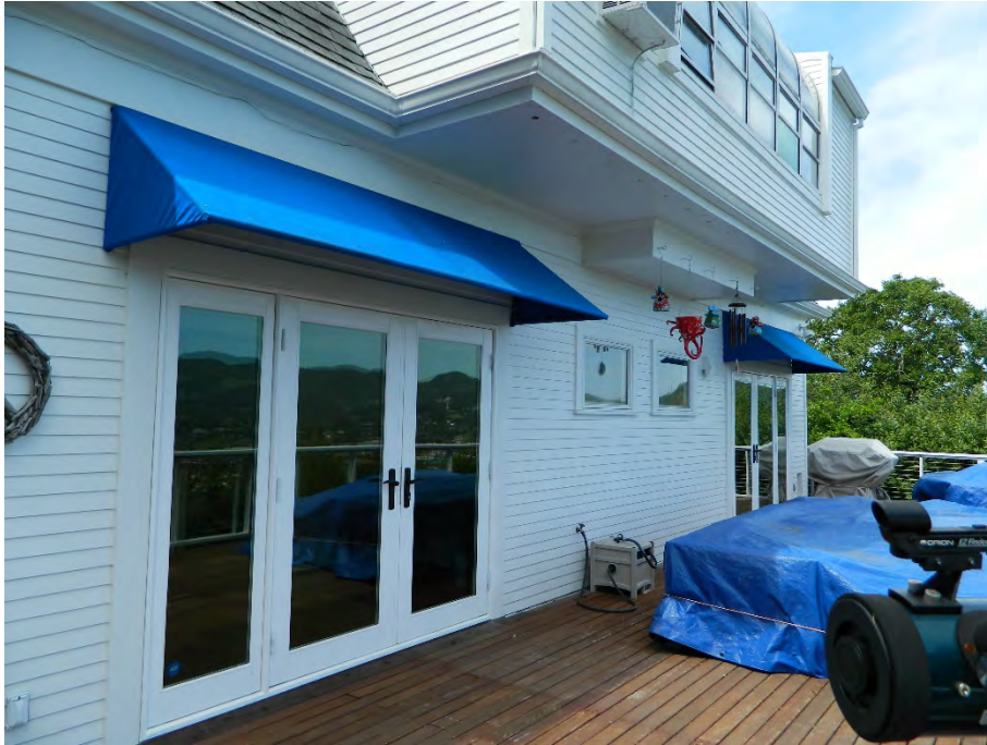
Photo showing the first story, facing north/northwest. Doors, windows, and second-story addition appear to be modern.
