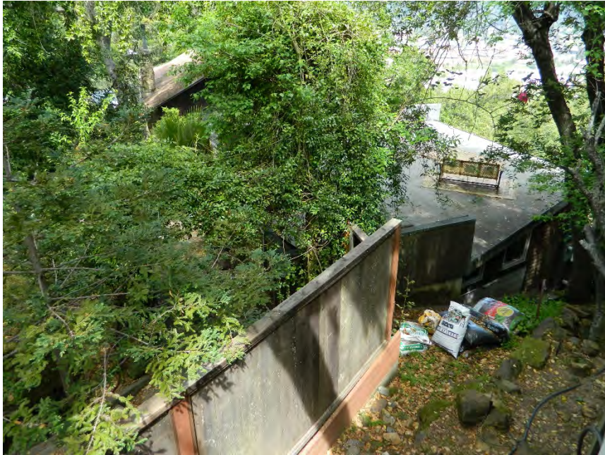
Photo showing the south elevation, facing north/northeast.
