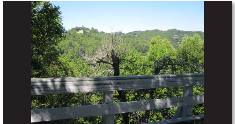
View from western edge of bridge, facing west.
