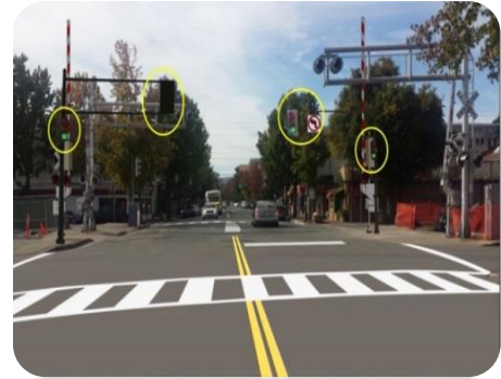
Queue Cutters recently installed at a SMART rail crossing on 4 th Street
