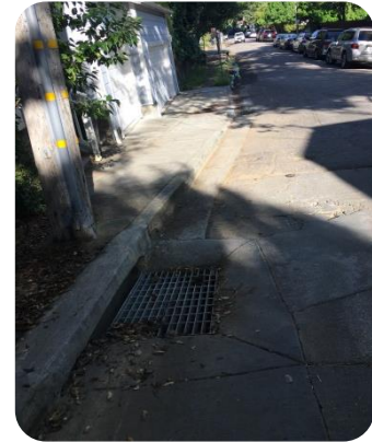
Curb and gutter at East and Jessup
