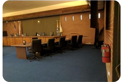
Fire extinguisher in the City Hall Council Chambers
