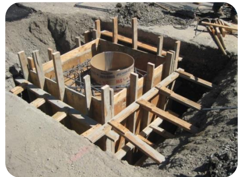
Example of grout work
