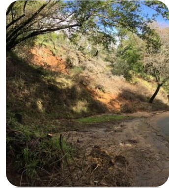
76 D Street hillside damage
