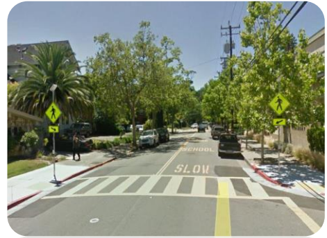
Mid-block crossing with flashing signs
