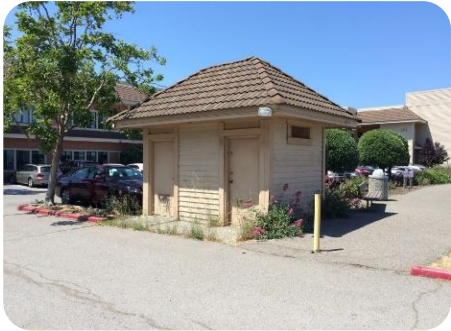
Current closed bathroom at Shoreline Park
