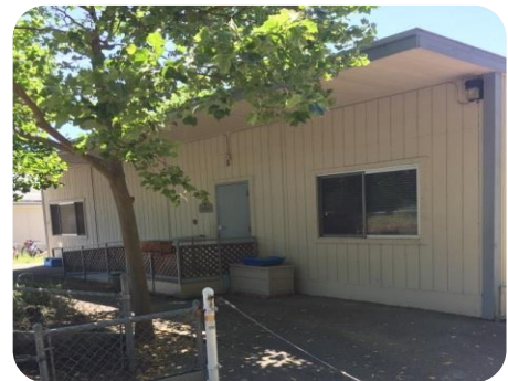
Portable building to be replaced at Dixie
