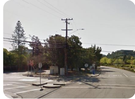
Example of overhead utilities
