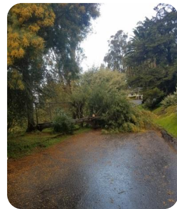
Fallen tree during winter storm
