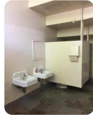
Current conditions of Albert Park Ball Field Restrooms
