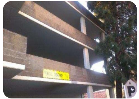
3 rd and A parking structure
