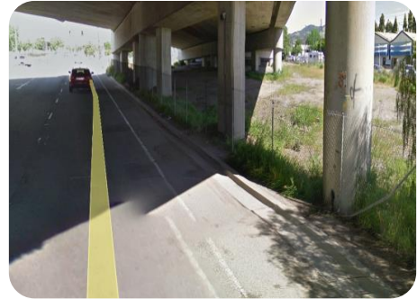
Bellam Blvd under the Highway 101 overpass
