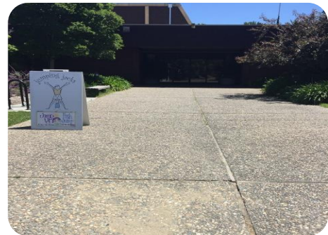
Concrete patio facing front entrance
