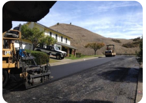
Street resurfacing work
