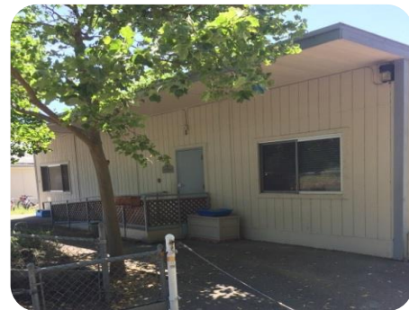
Portable building to be replaced at Dixie
