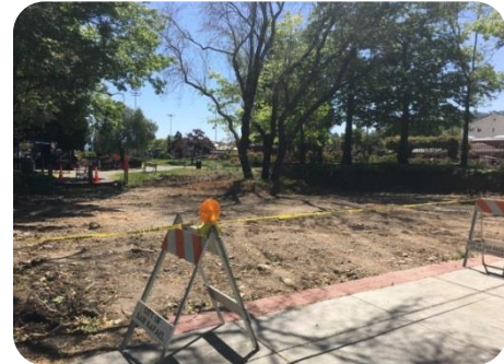
Albert Park Construction
