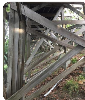
Southern Heights Bridge
