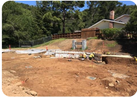
Current construction at Victor Jones
