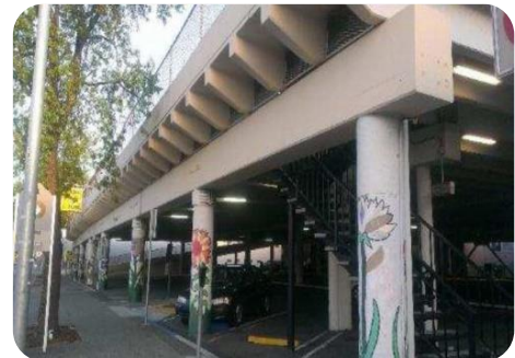
3 rd and Lootens parking structure
