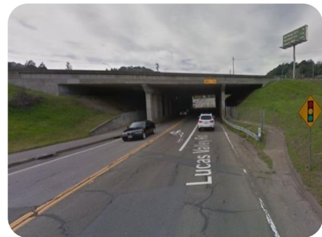
Smith Ranch Road under Highway 101
