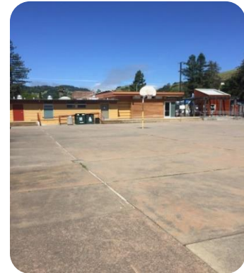
Pavement in the B Street Parking lot
