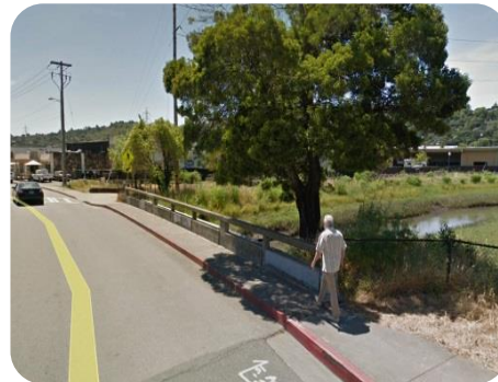
Lincoln Avenue Bridge
