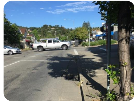
Curb and drainage on 2 nd Street
