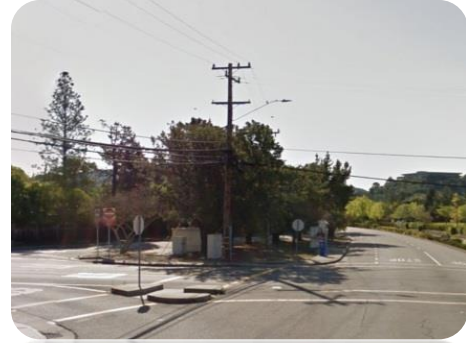
Example of overhead utilities
