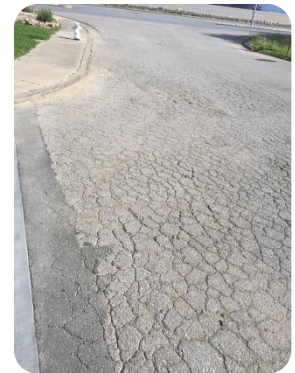
Driveway and parking lot at Fire Station 55
