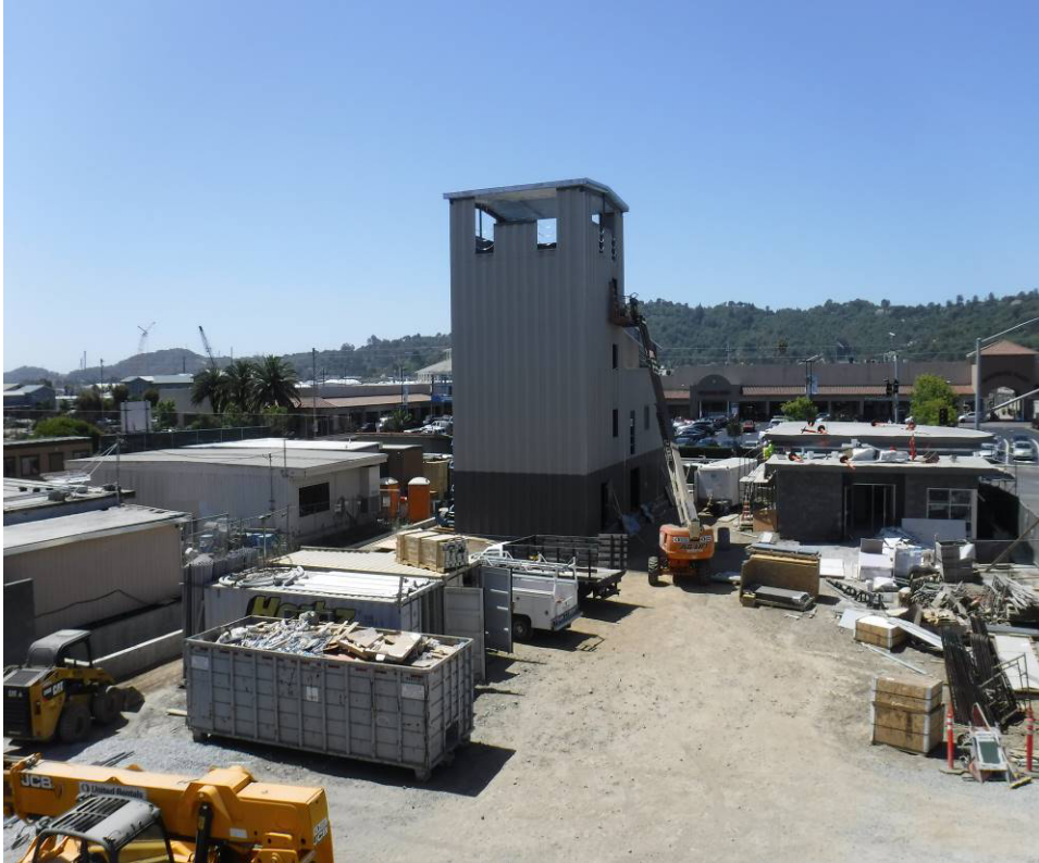
June 2018 progress pictures for Fire Station 52
