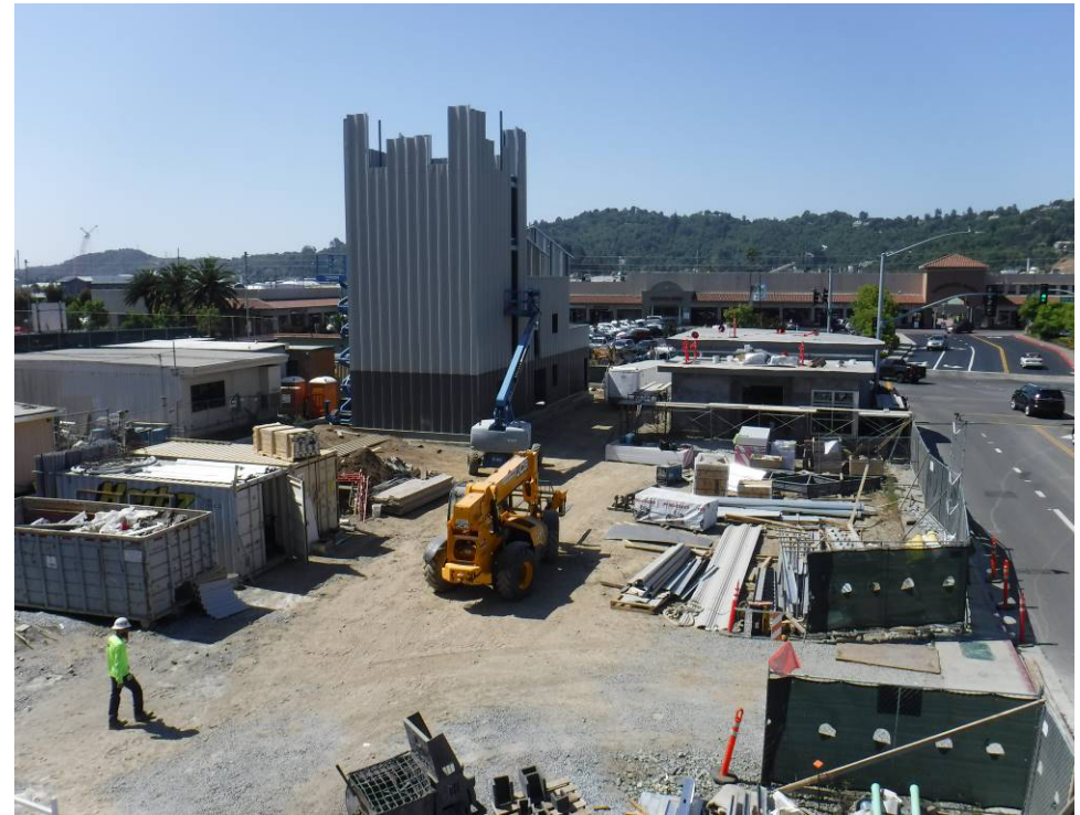
June 2018 progress pictures for Fire Station 52
