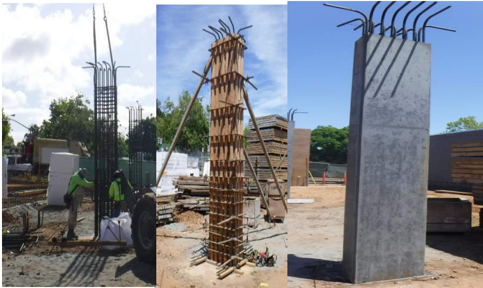
June progress picture – Column being erected formed and stripped.
