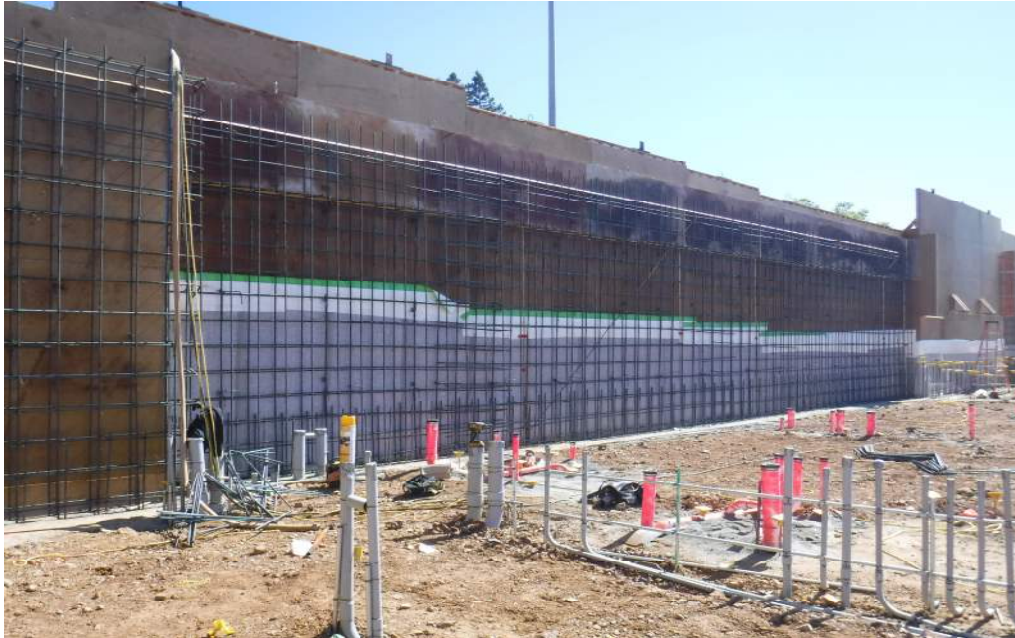
June progress pictures – Shotcrete forms, waterproofing and rebar installed
