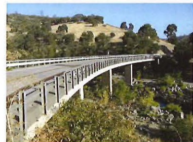
Amador County Consumes River Bridge at Lathrobe Road—Construction Management performed by Coastland
