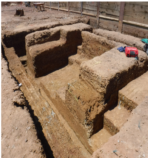
May progress picture – excavation of footing and elevator pits
