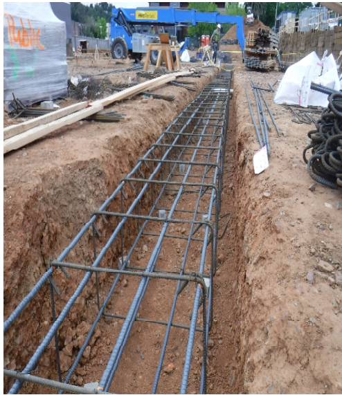
May progress pictures – installation of rebar and conduits
