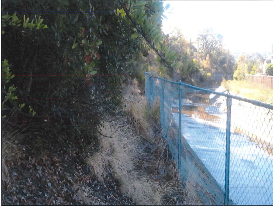
Photo 3. West side of the site showing patch of native grassland, chain-link fence, and Gallinas Creek.
