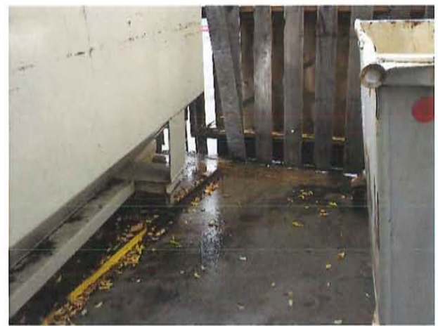
12. Garbage-Related Liquid Releases from Trash Compactor Unit
