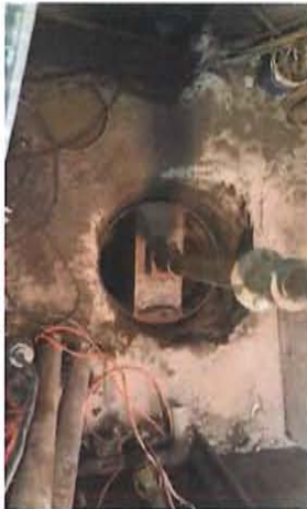
27. Augur bit used to enlarge and straighten elevator #3 jack hole
