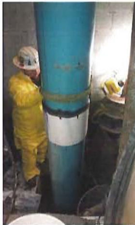
33. PVC secondary casing being installed into elevator jack hole
