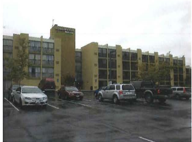
2. Southeastern Façade of East Tower
