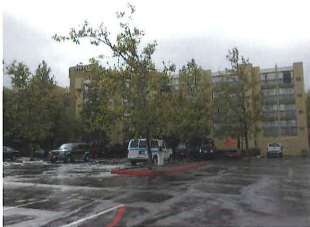
3. Northern Façade of North Tower and Northern Parking Lot
