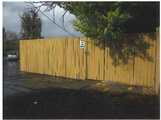
10. Exterior Trash Compactor/Dumpster Enclosure
