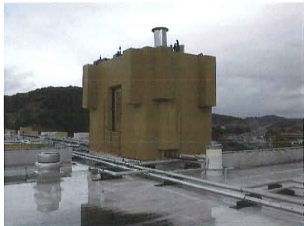
18. North Tower Roof, View Facing North
