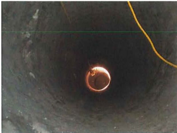
31. Bottom of jack hole. Notice scoured side walls and absence of groundwater.
