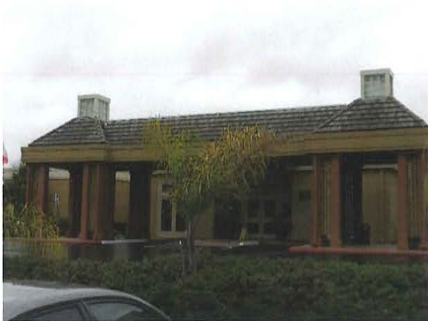
1. Southwestern Facade of Front-of-House/Conference Center Building
