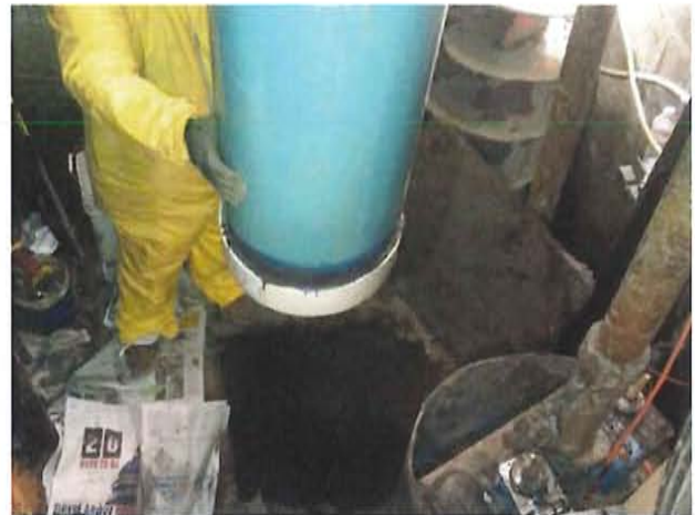
32. PVC secondary casing being installed into elevator jack hole
