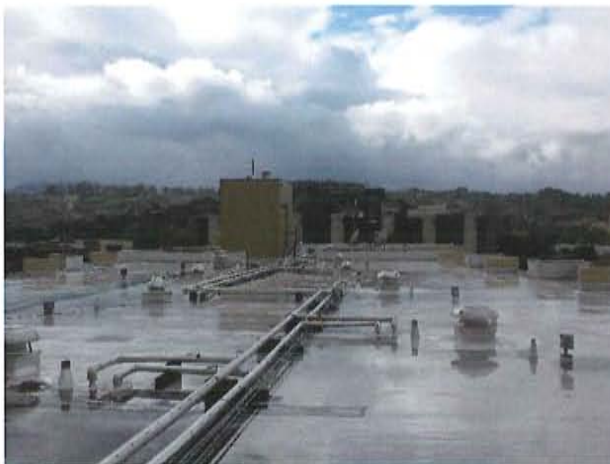
17. East Tower Roof, View Facing Southwest
