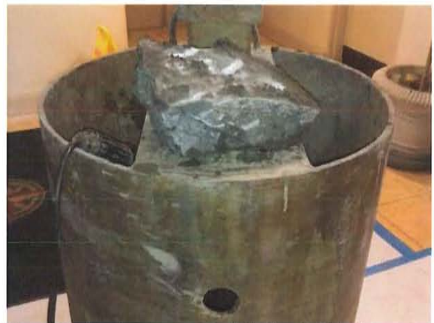
30. Bedrock encountered during jack hole enlargement
