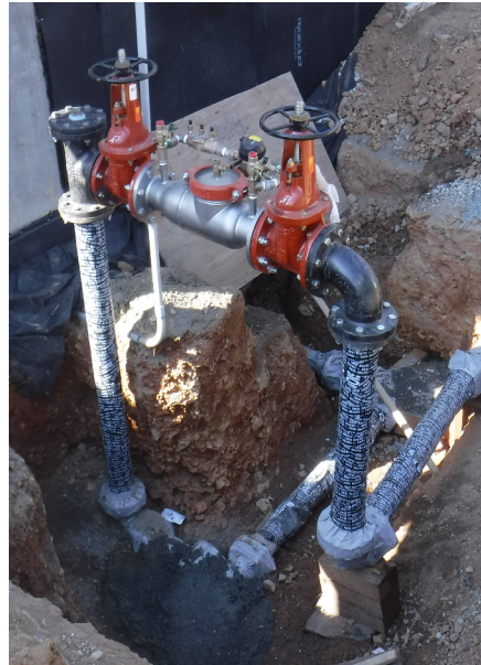
October progress pictures—Domestic Water connection on the left / Fire Backflow valves on the right
