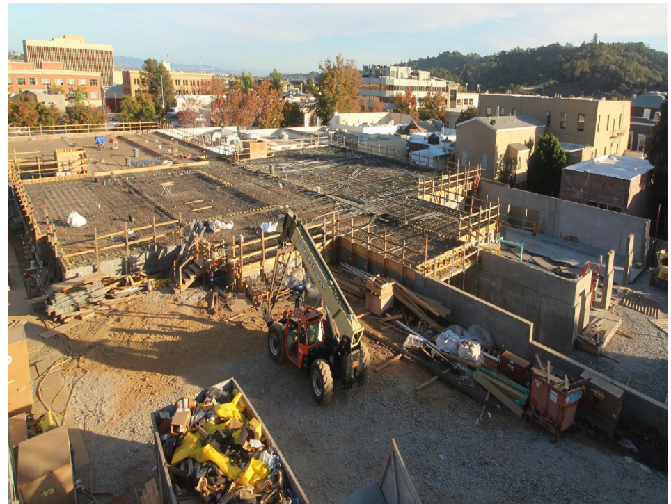
October progress picture – Overview of project site progress.
