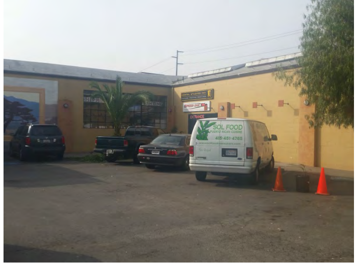
2. Subject property parking lot followed by the main entrance into Flemming Tax Service and Dostal Studio Inc.
