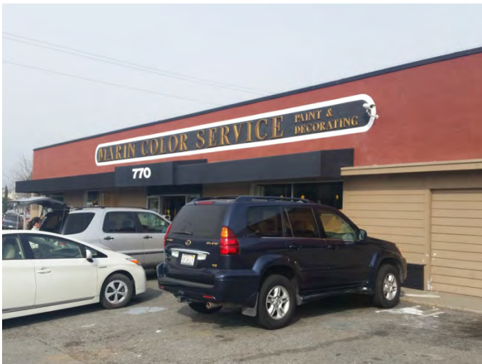
19. Southern adjacent Marin Color Service (770 2 nd Street) formerly a gas station and noted in the regulatory database (refer to Section 5.1)
