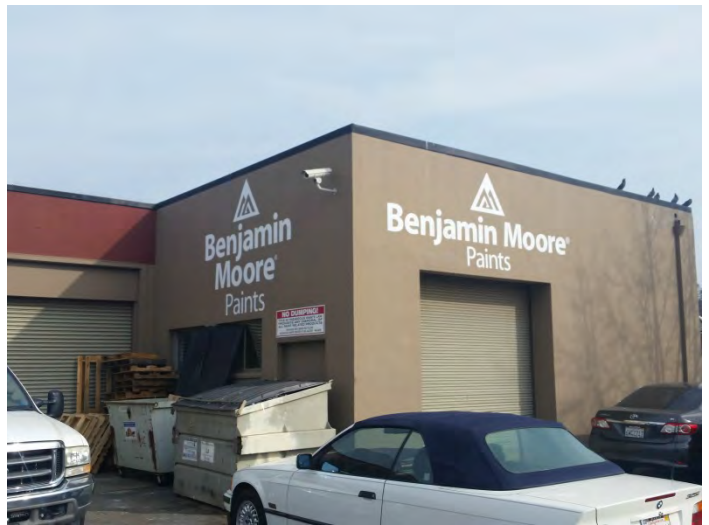
20. Additional portion of the Southern adjacent Marin Color Service (770 2 nd Street)
