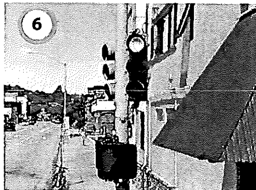
Intersections without mast arms and without 12" LED signal heads have lower visibility and can result in vehicles not being able to stop in time for a signal change
