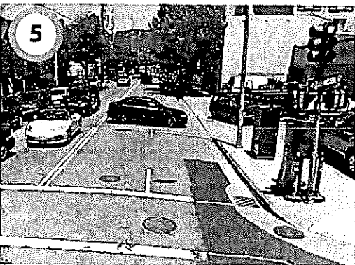
Intersections throughout the Third Street Corridor lack mast arms which can diminish visibility and clarity of signals
