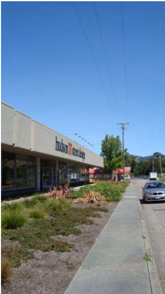
1-story Hudson Design building on Redwood Highway
