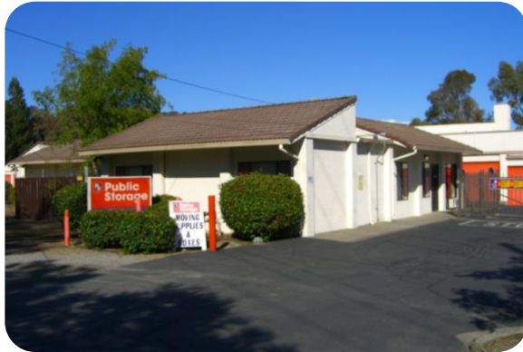
Public Storage on Merrydale Road
