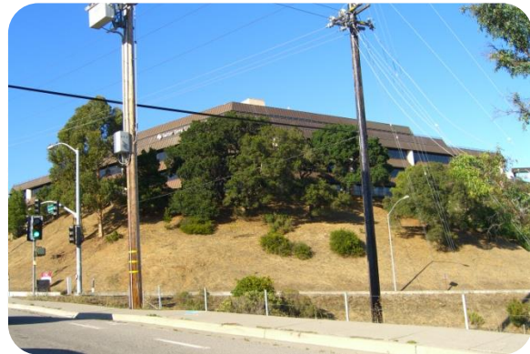
Sutter Terra Linda Urgent Care Facility
