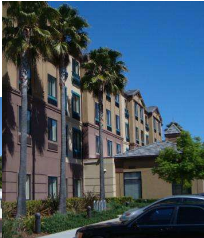
4-story Extended Stay hotel building
