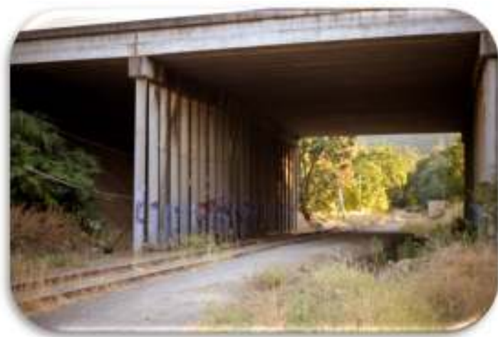
EXHIBIT 3-9 Rail undercrossing of US101
