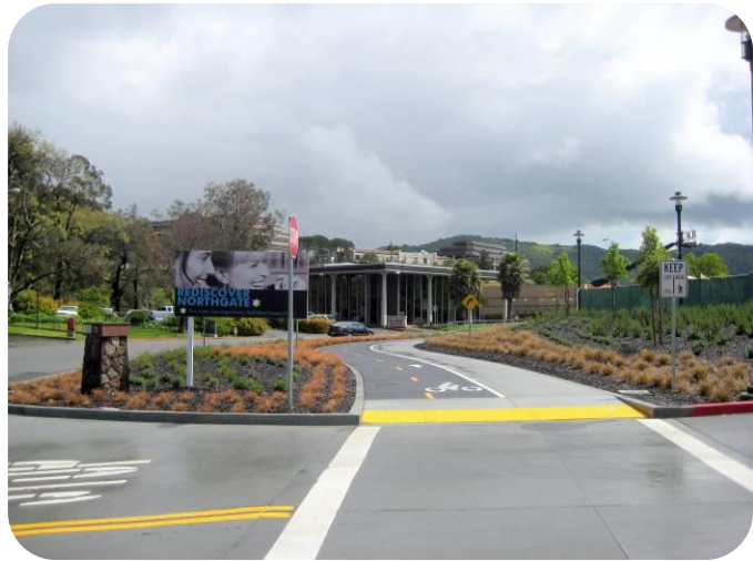
The North San Rafael Promenade should be extended to connect with the Civic Center Station
