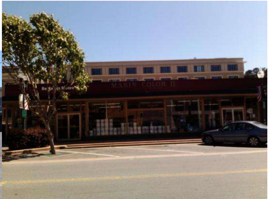
4-story Whole Foods building, Novato, in background, rising above the Marin Color building in the foreground
