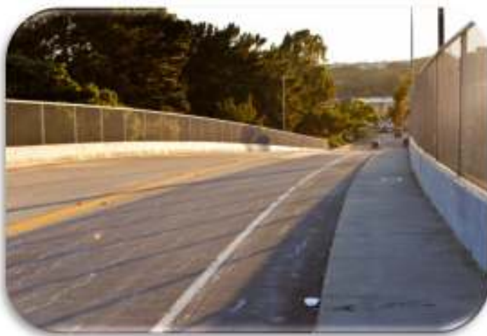
EXHIBIT 3-3 Merrydale Overcrossing looking west
