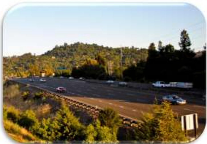
EXHIBIT 3-1 US101 looking south
