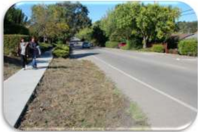
EXHIBIT 3-4 Los Ranchitos Road looking north
