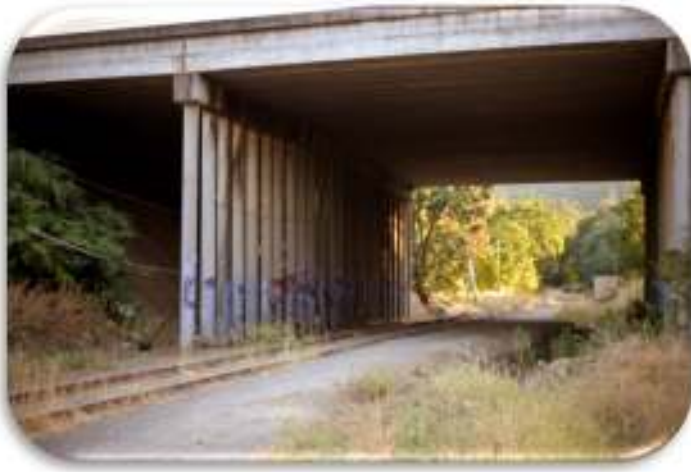
EXHIBIT 3-9 Rail undercrossing of US101
