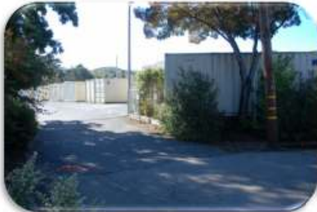
EXHIBIT 2-8 The Northgate Storage facility on Merrydale Road north of the railroad tracks
