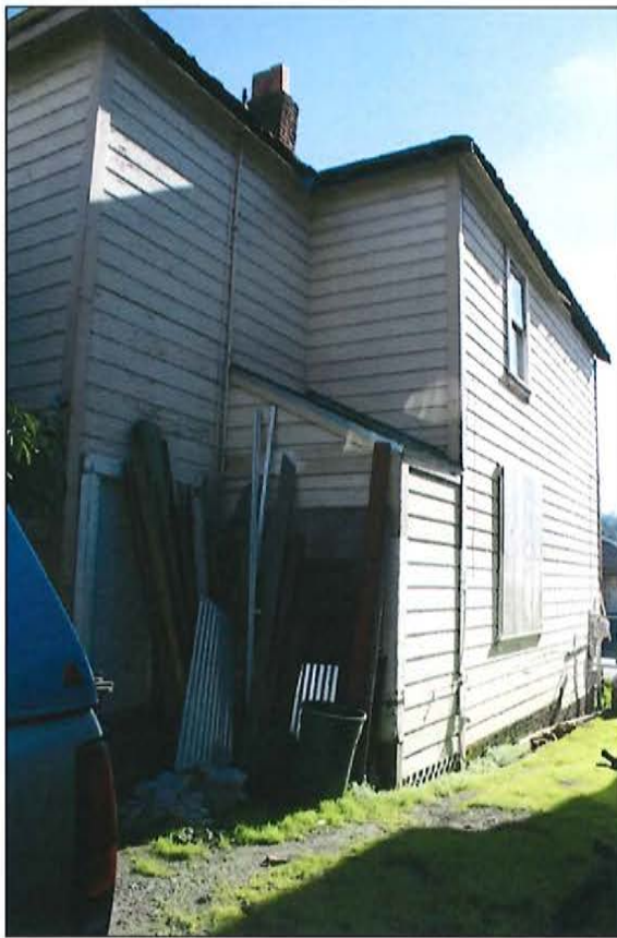
West side façade, looking southeast
