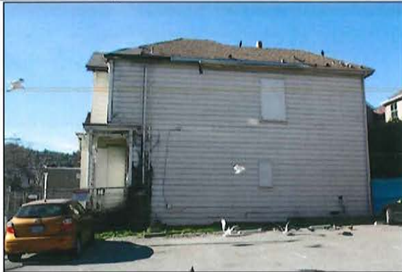
East side façade
