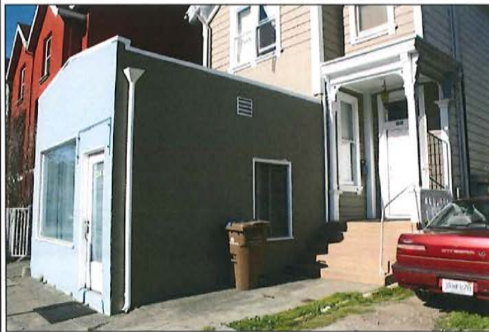
Front (south) façade showing entry
