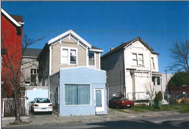
Setting – front facades of 1212 & 1214 2 nd
