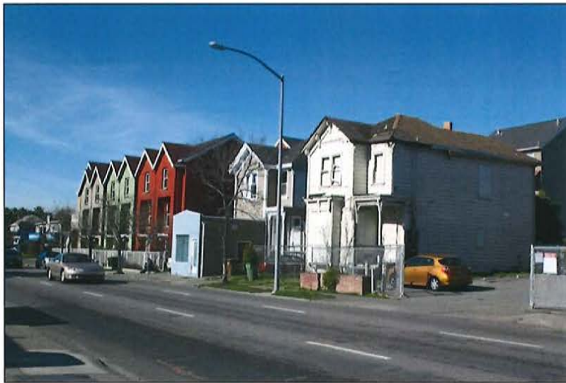
Setting – east side facades of 1212 & 1214 2 nd
