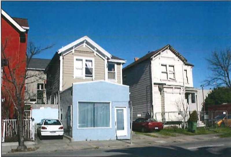
Setting – front facades of 1212 & 1214 2 nd
