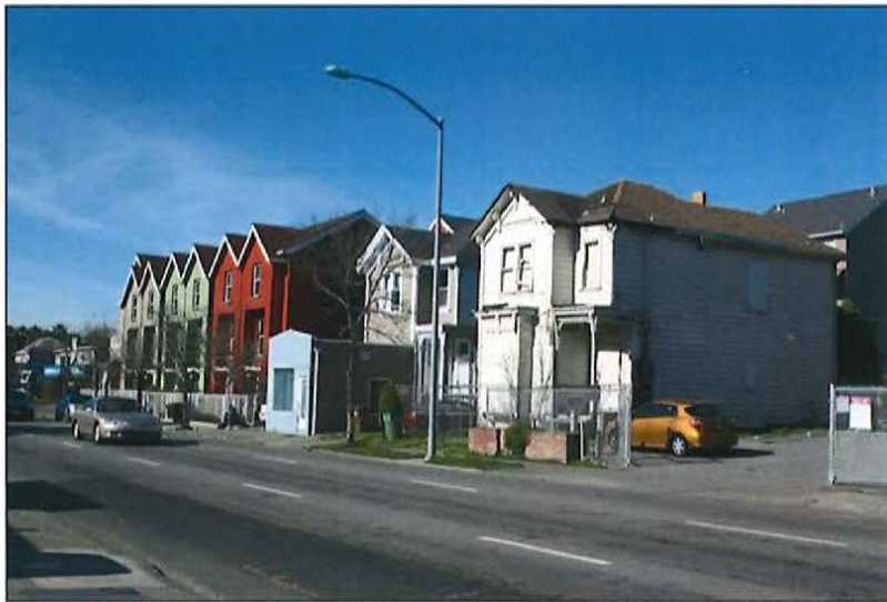
Setting – east side facades of 1212 & 1214 2 nd
