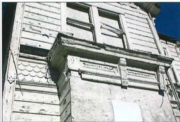
Detail of front facade
