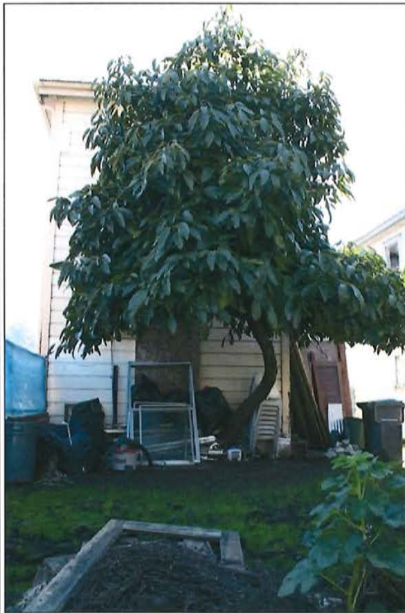
North rear facade
