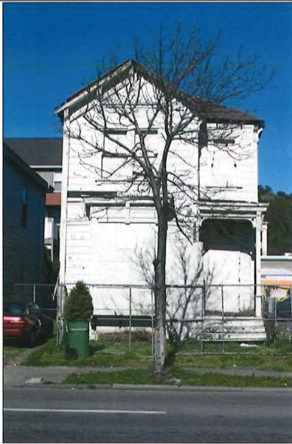
Front (south) façade
