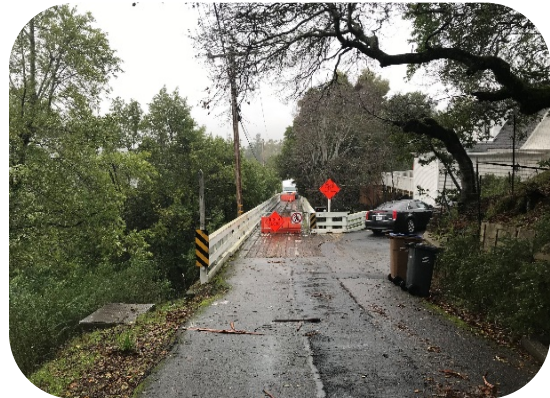
Beginning of the bridge from Meyer Road
