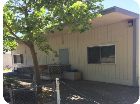
Portable building to be replaced at Dixie
