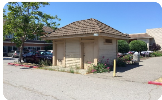
Current closed bathroom at Shoreline Park
