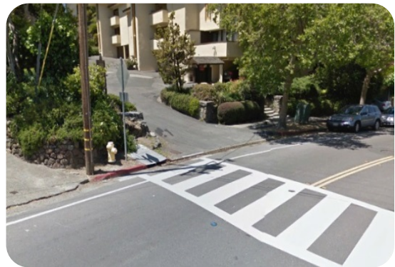
201 D Street Crosswalk
