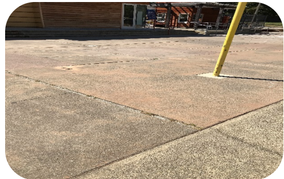
Terra Linda Community Center Basketball Court
