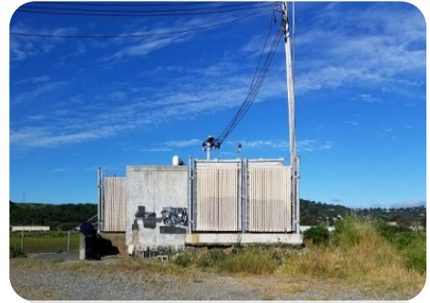
San Quentin Pump Station
