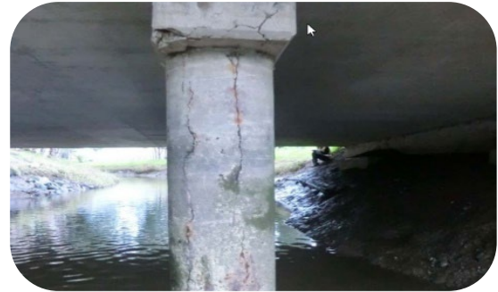
Detoriated substructure
