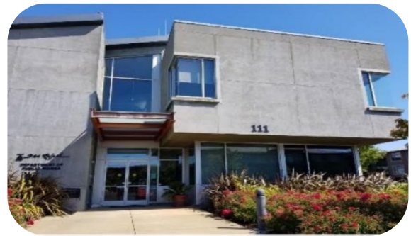
Department of Public Works Offices
