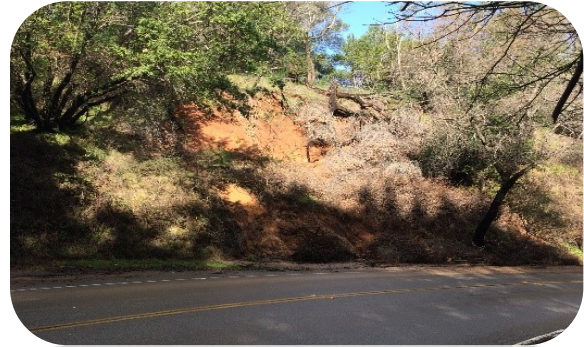
76 D Street Hillside Damage
