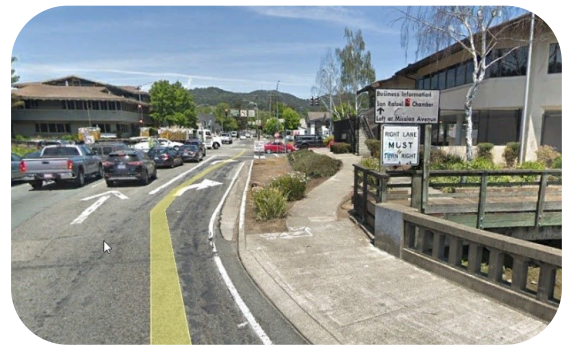
Right-turn lane from Northbound 101 to Second Street
