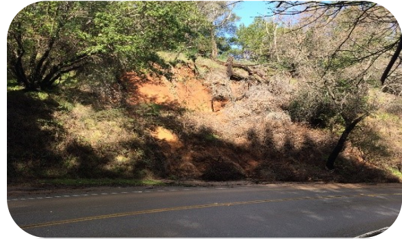
76 D Street Hillside Damage
