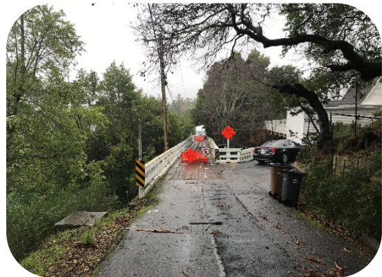
Beginning of the bridge from Meyer Road
