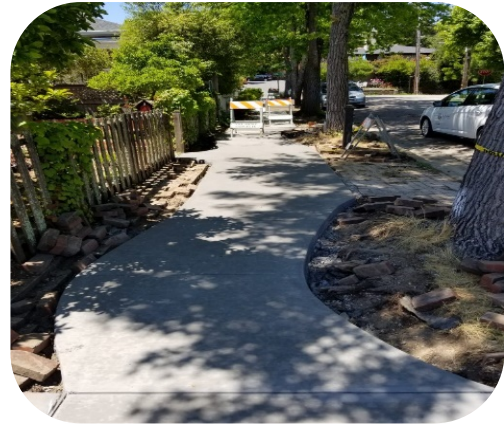
Bayview St. repaired by constructing the sidewalk around the tree
