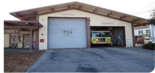
Front of Fire Station 54
