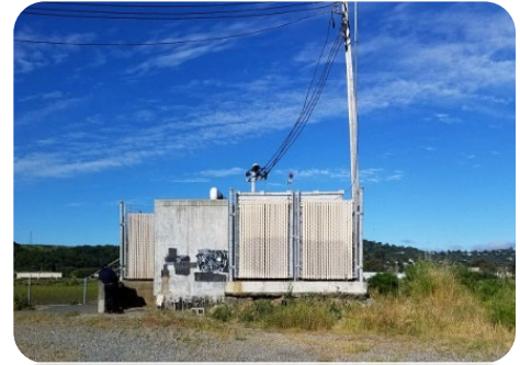
San Quentin Pump Station
