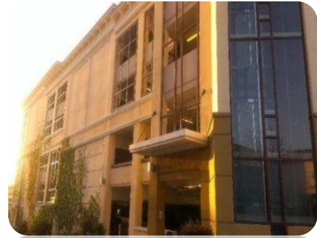
Third and C Parking Structure
