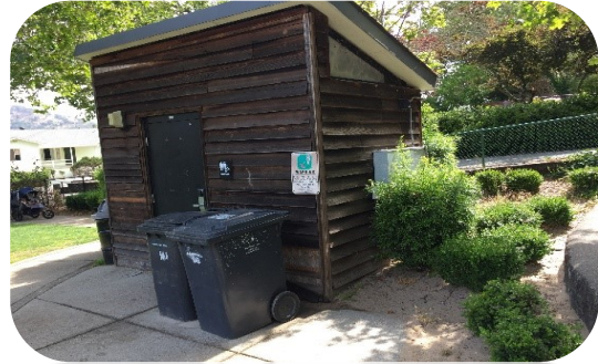
Gerstle Park Restroom
