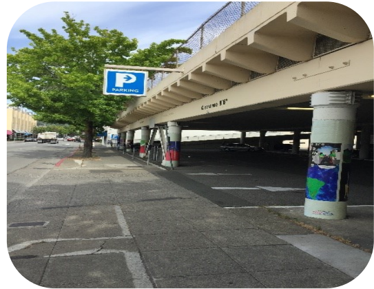
Third and Lootens Parking Structure
