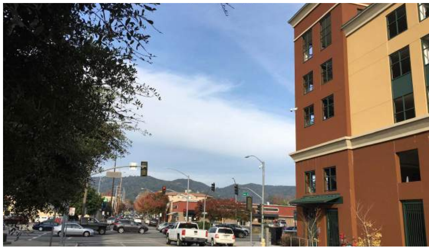
3 VIEW FROM LINCOLN AVENUE LOOKING TOWARDS 2ND STREET
