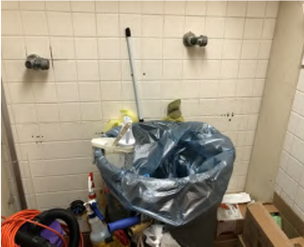
2.2 Level 1 Staff men's restroom
