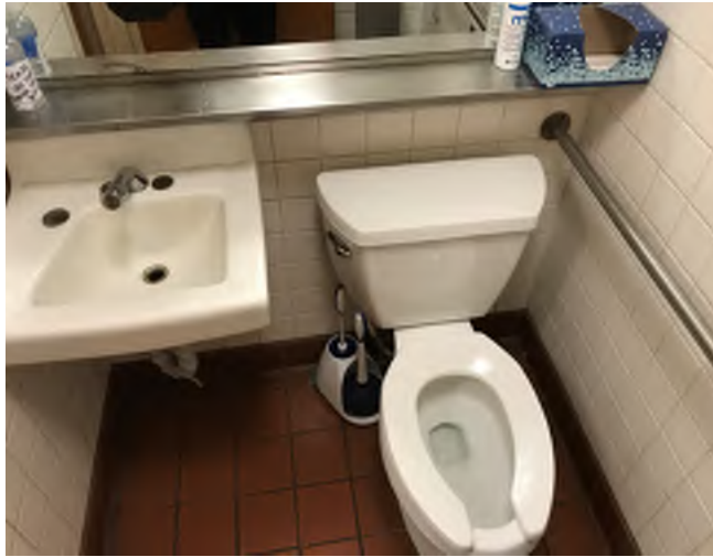
2.4 Level 1 Staff women's restroom
