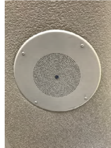
9. Example of a typical IP Speaker (if used in renovation)
