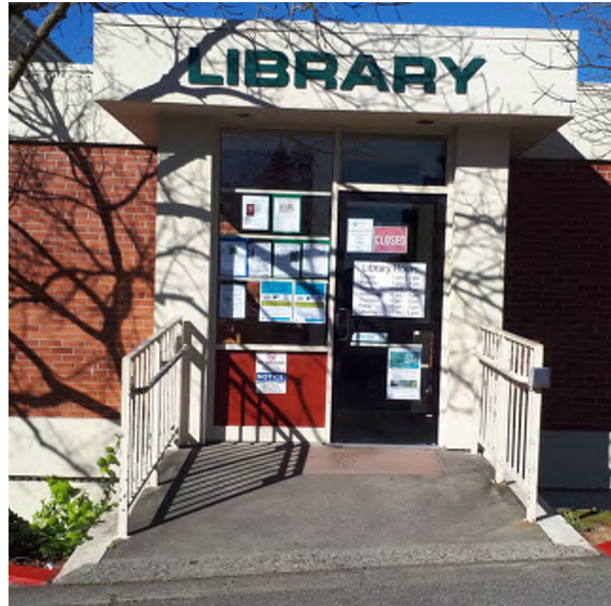
Existing landing on east Entry
