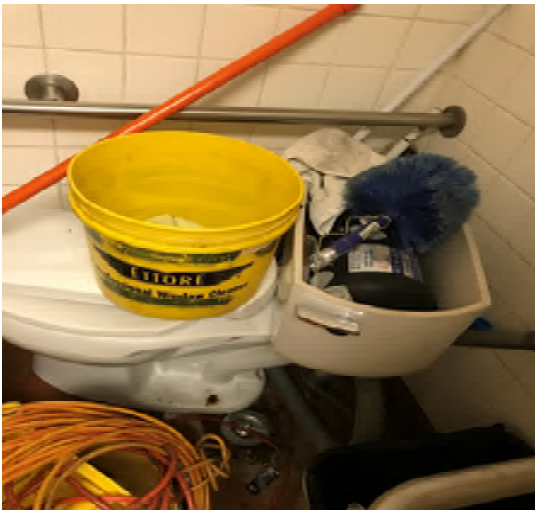
2.1 Level 1 Staff men's restroom
