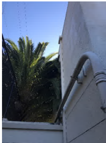
Exterior Feeder to Old Service
