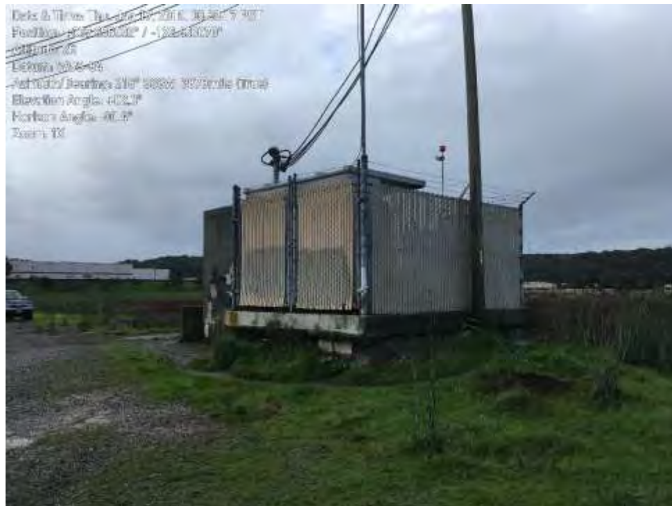
TH000069, view southwest, 1/17/2019: View of the northeast corner of pump station.
