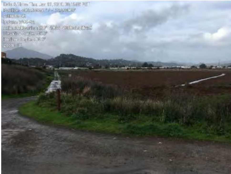
TH000079, view west, 1/17/2019: Overview of access road which covers storm drain pipe.
