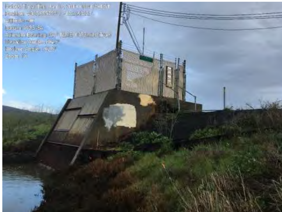
TH000073, view northeast, 1/17/2019: view of the southwest corner of the pump station.
