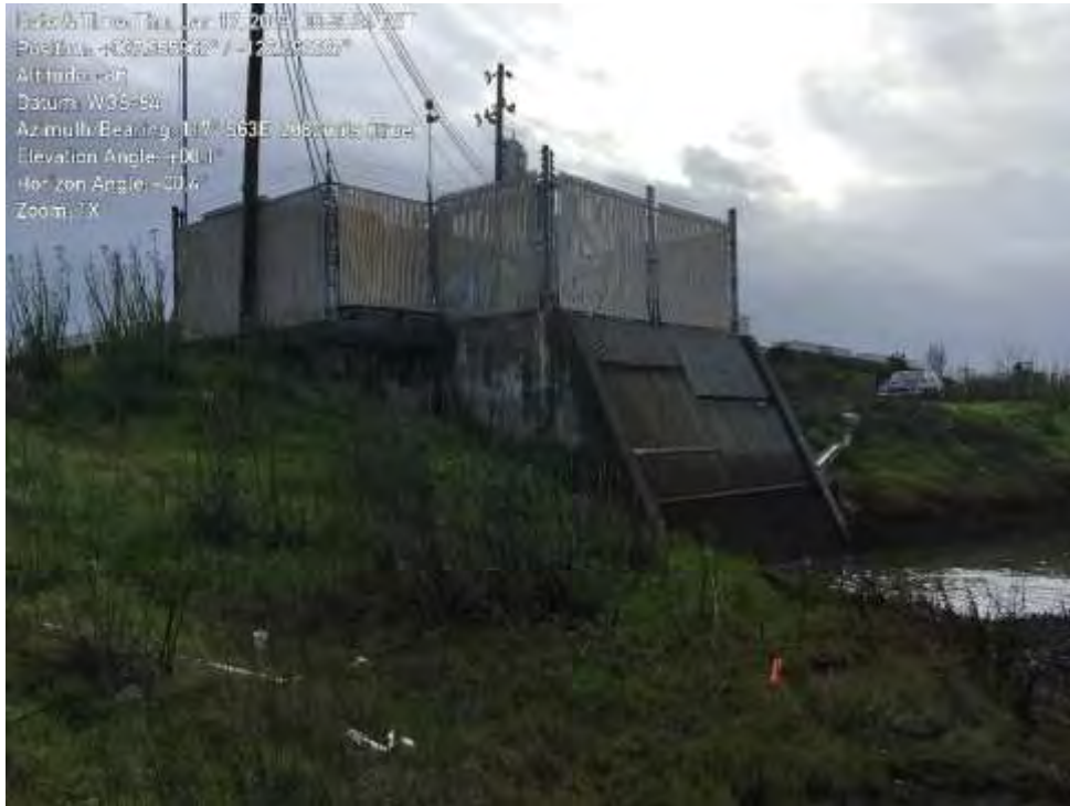
TH000071, view southeast, 1/17/2019: View of northwest corner of pump station.
