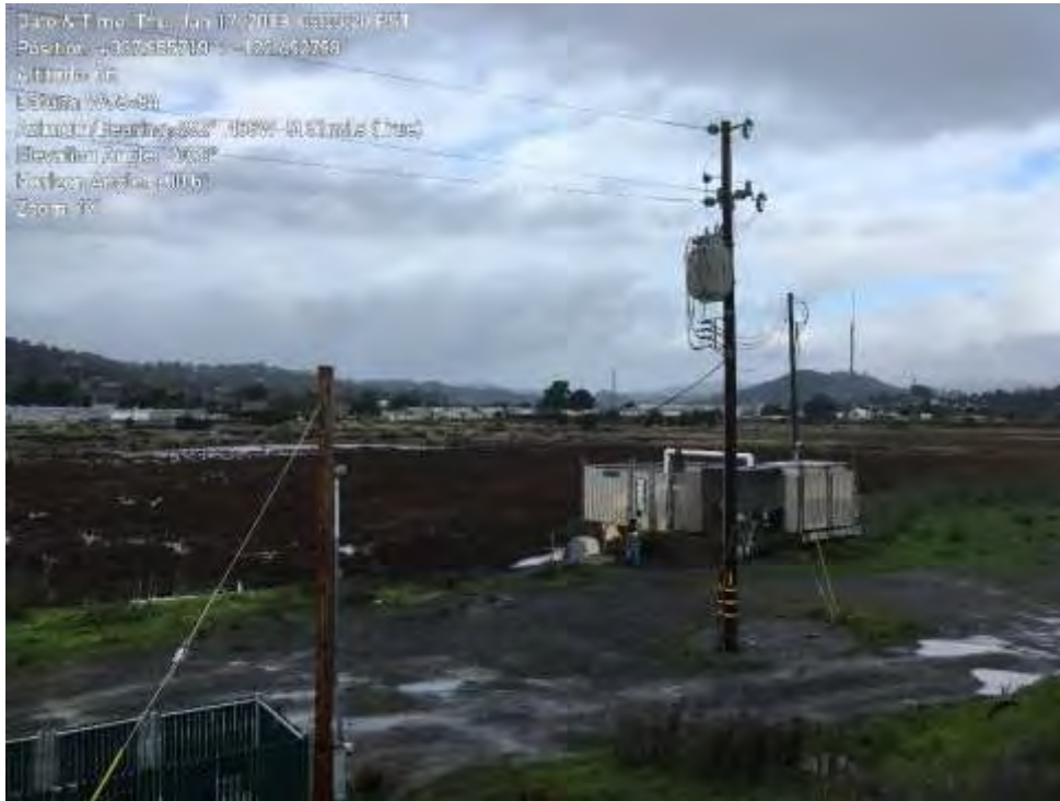
TH000075, view northwest, 1/17/2019: Overview of pump station, utility pole and lagoon.
