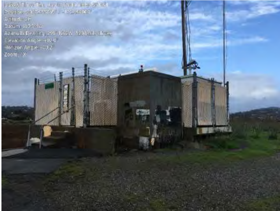
TH000067, view northwest, 1/17/2019: View of the southeast corner of pump station.
