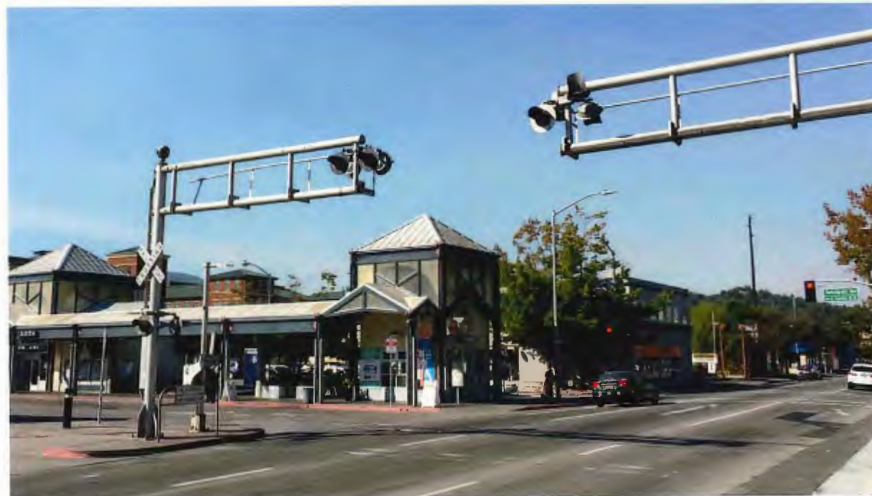
2 VIEW DOWN 3RD STREET FROM TRANSIT CENTER
