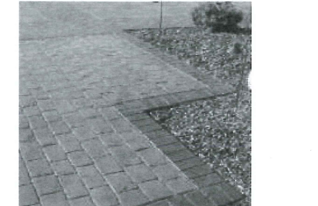
ENHANCED PAVING AT CROSSWALKS COLORED / STAMPED CONCRETE
