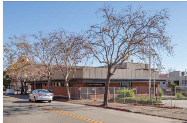
4 LOOKING EAST ON 5TH AVENUE
