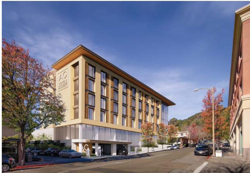
VIEW LOOKING NORTH FROM B STREET
