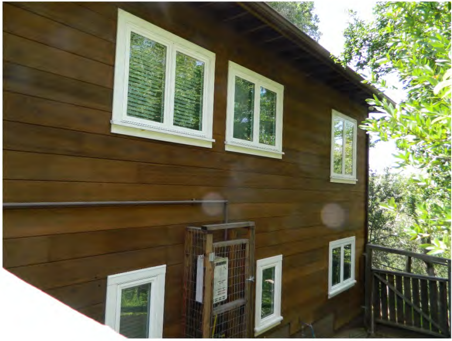
Photo showing the northeast elevation, facing west.
