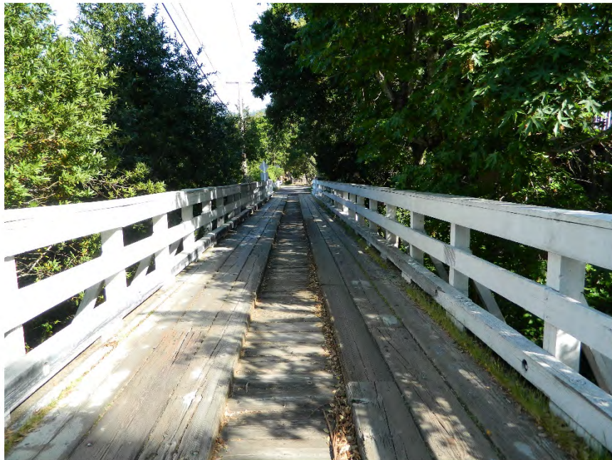
Photo showing the north approach to the bridge, facing south.
