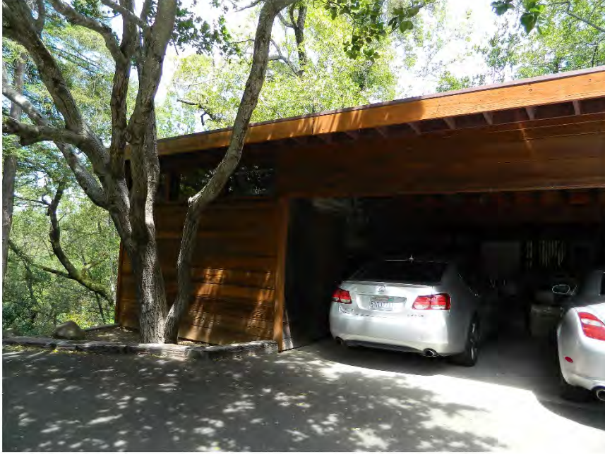
Photo showing the carport, facing north.
