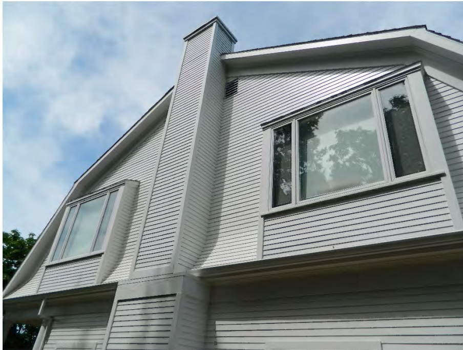
Photo showing the south elevation, facing north/northwest.
