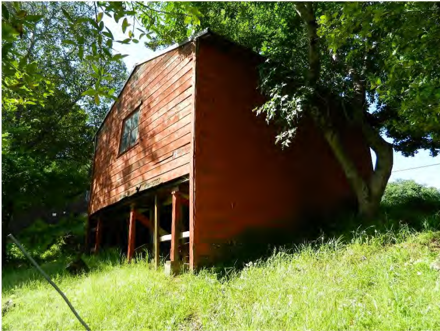
Photo showing the east and north elevation, facing south.
