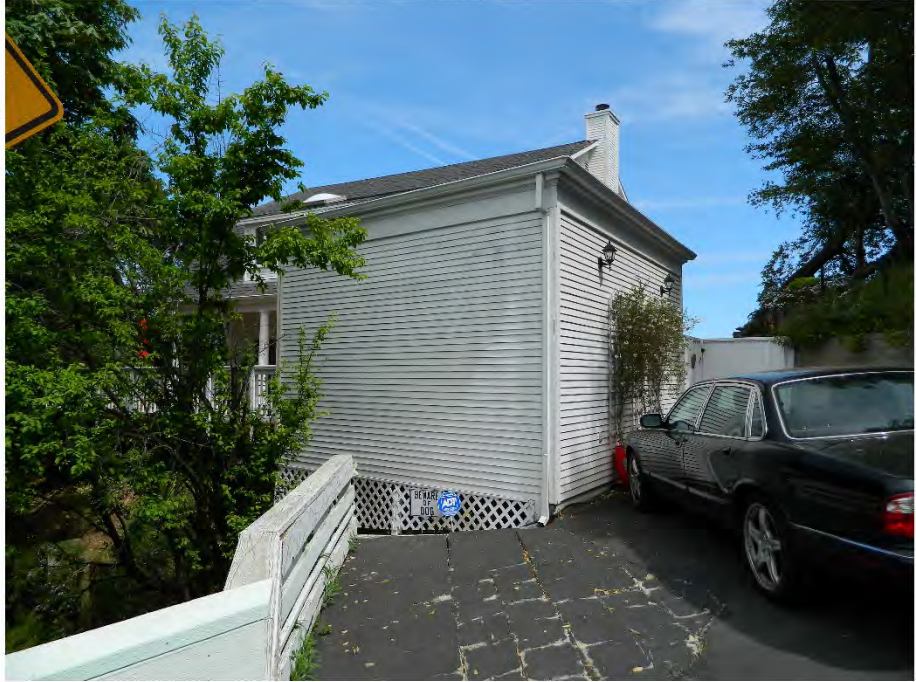
Photo showing accessory building, facing north/northwest.
