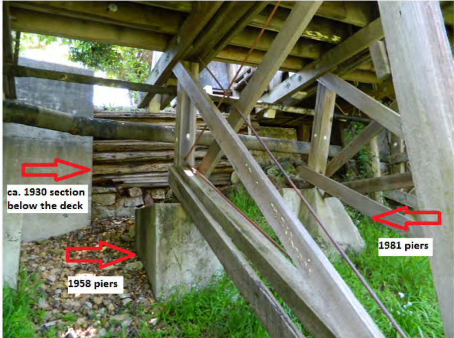
Photo showing the supporting membranes of the bridge, facing east.
