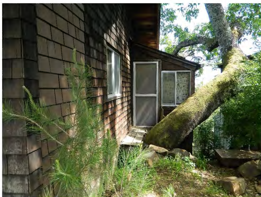
Photo showing the south elevation, facing west.
