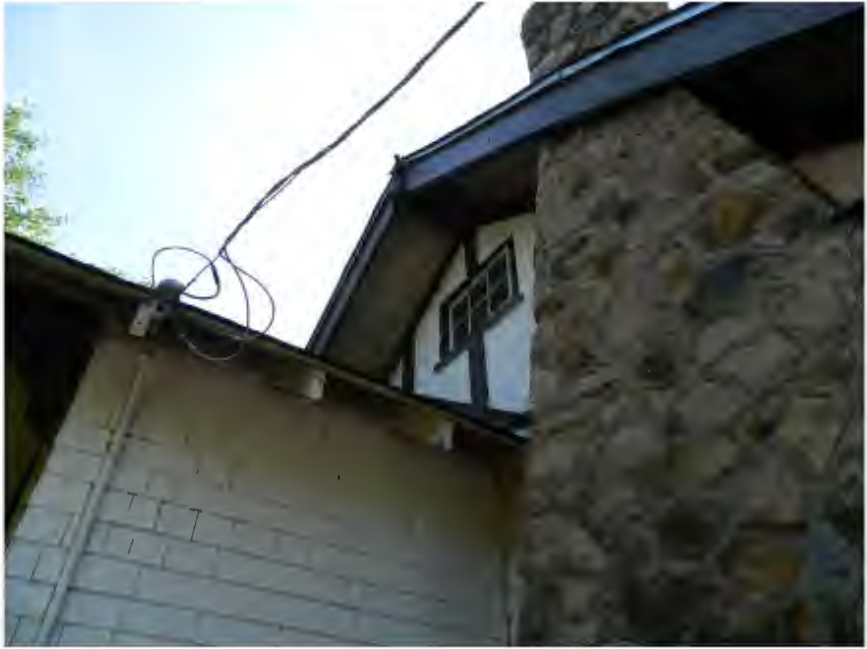
Photo showing the north elevation second story, facing east.
