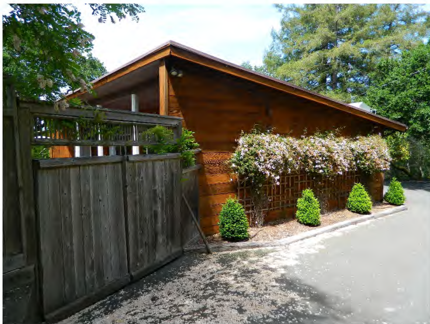
Photo showing the southeast elevation, facing north.
