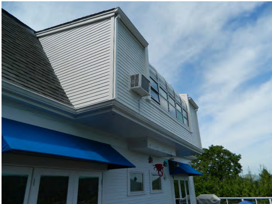
Photo showing the second story of the east elevation, facing north/northwest.
