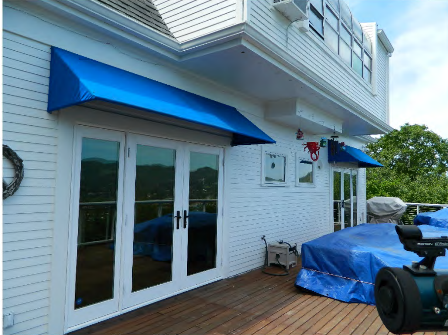
Photo showing the first story, facing north/northwest. Doors, windows, and second-story addition appear to be modern.
