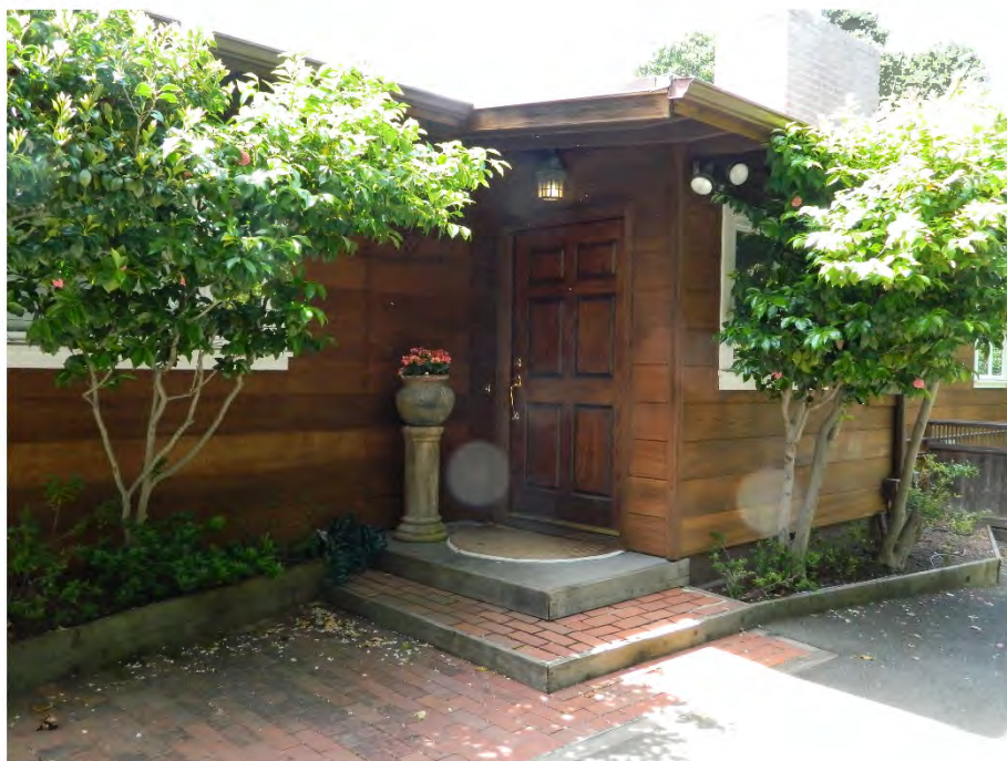
Photo showing the recessed front entry along the northeast elevation, facing southwest.
