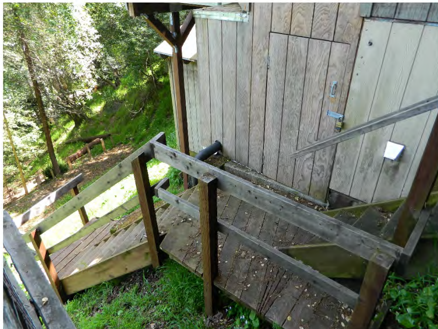
Photo showing the north elevation staircase, facing east/southeast.
