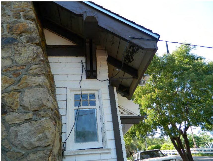
Photo showing the north elevation, and wooden knee braces.
