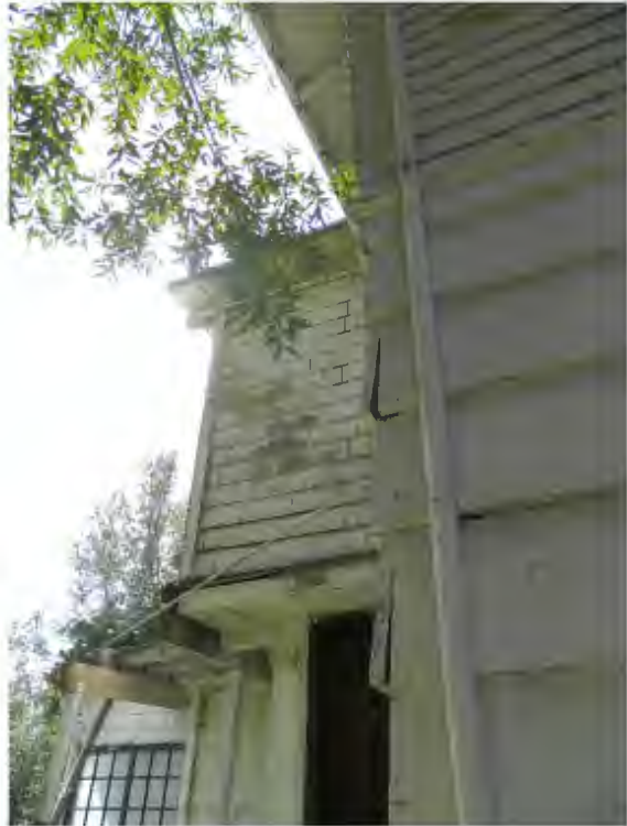
Photo showing the north elevation additions, facing south.
