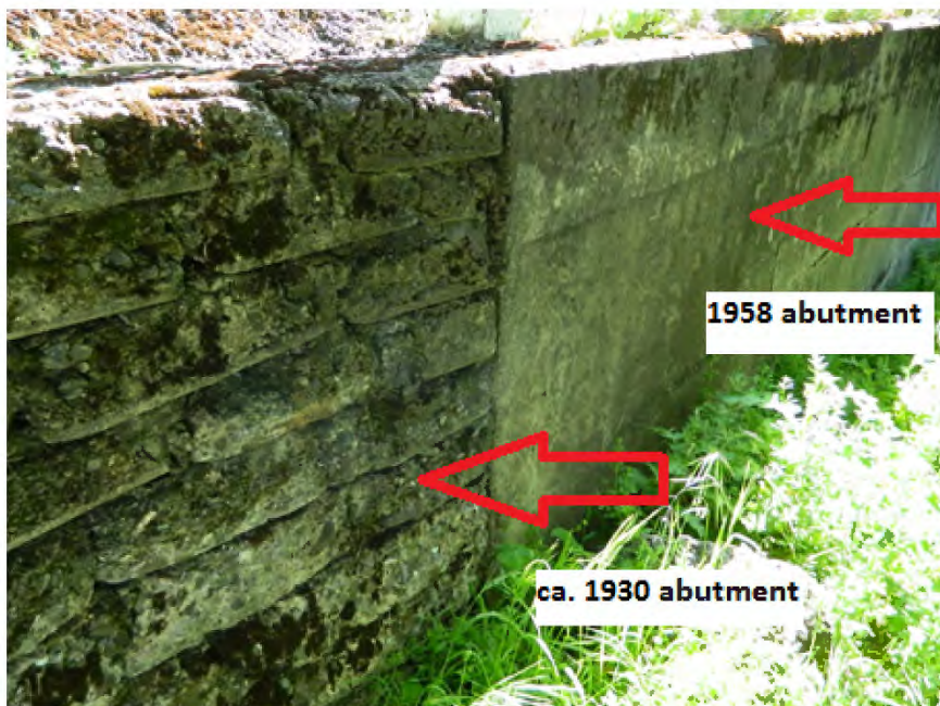
Photo showing ca. 1930 abutment and the 1958 abutment.
