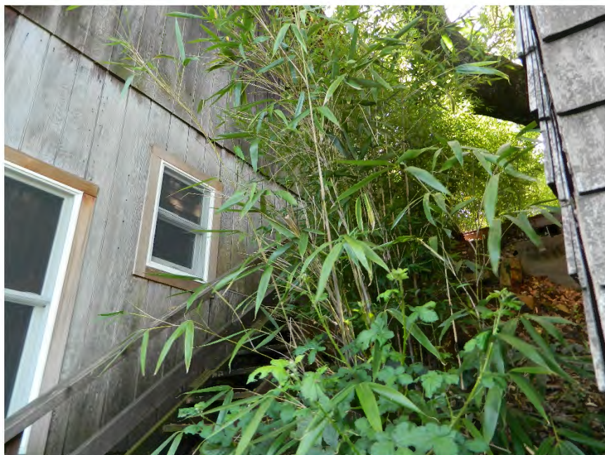
Photo showing the north elevation, facing west/southwest.
