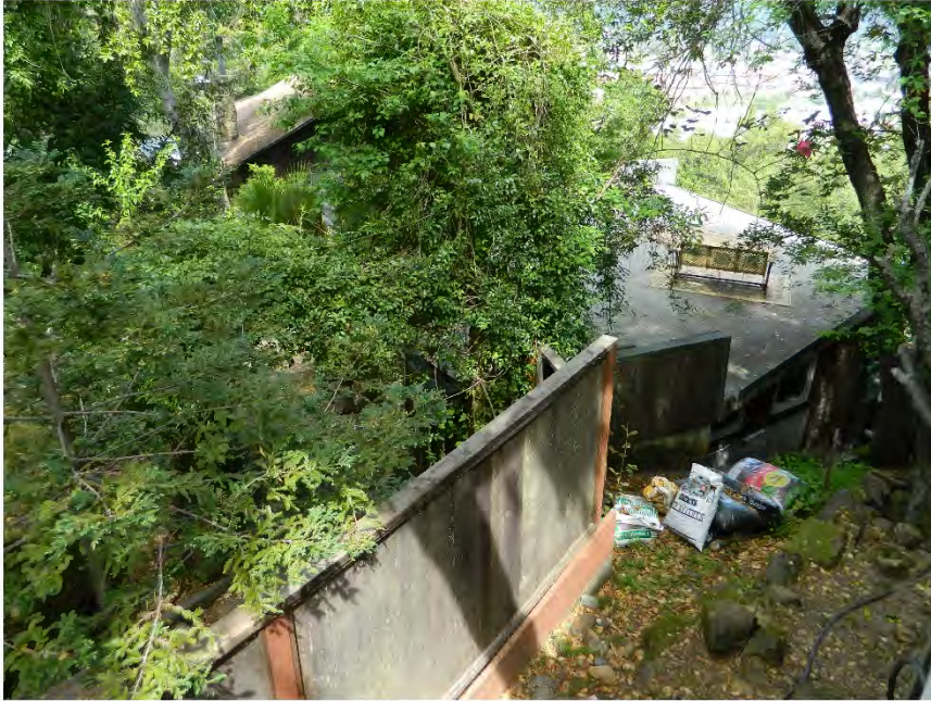
Photo showing the south elevation, facing north/northeast.
