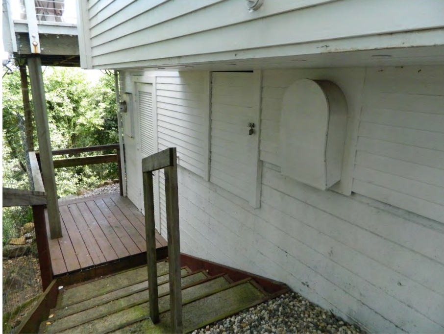
Photo showing the north elevation ground floor, facing southeast.
