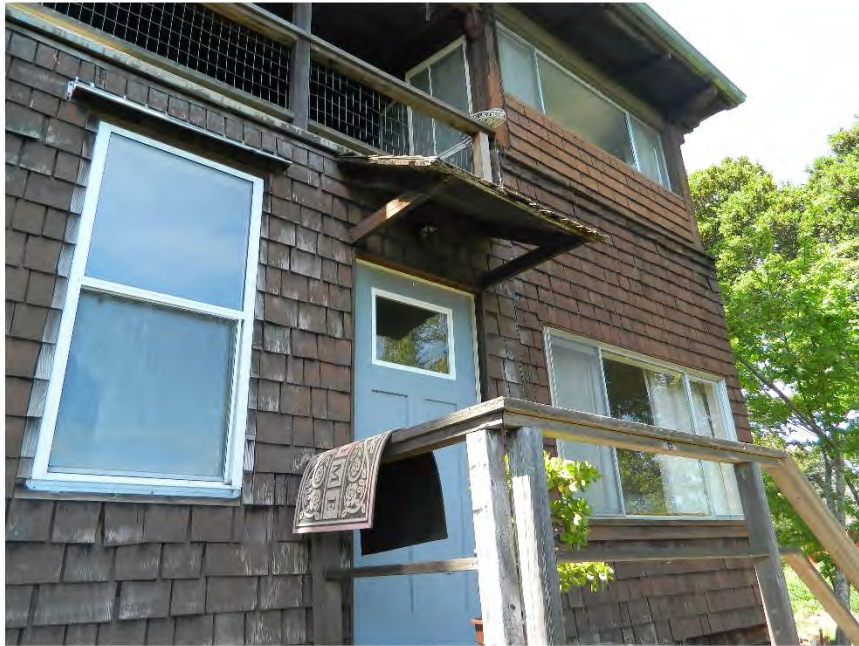
Photo showing the additions along the east elevation, facing west.
