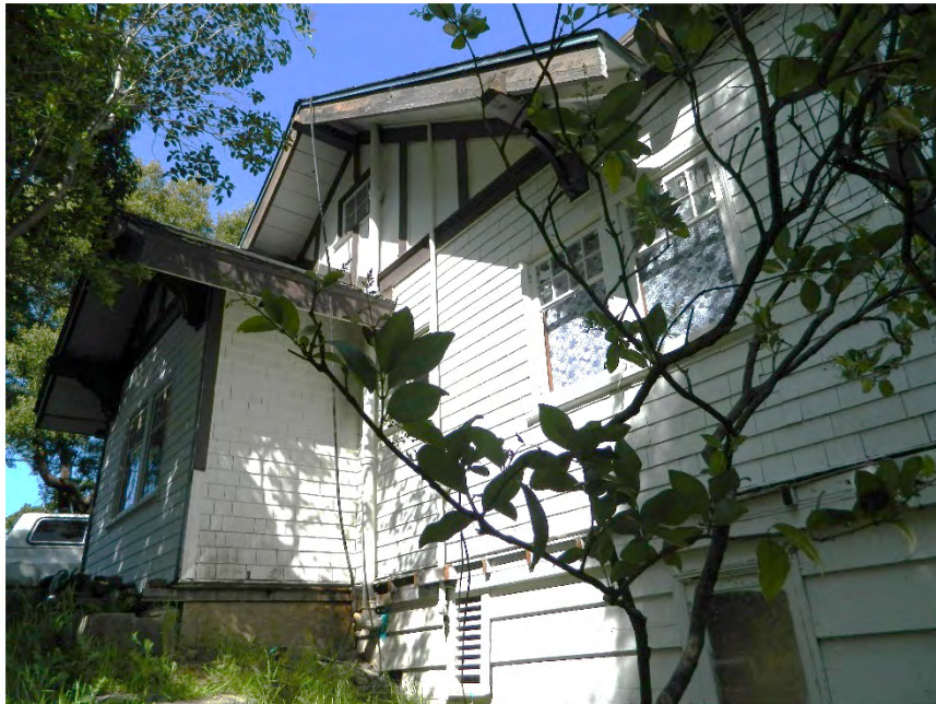
Photo showing the south elevation, facing north/northwest.
