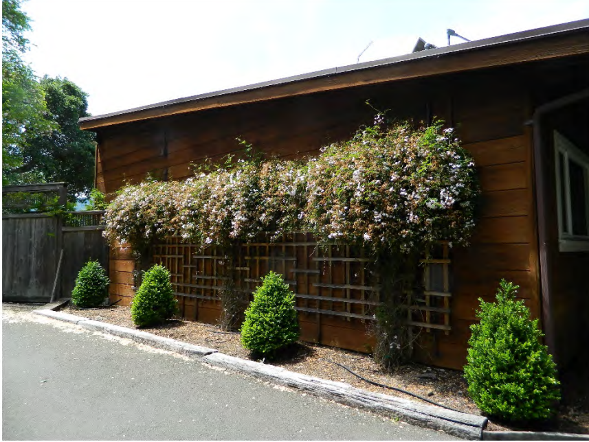
Photo showing the southeast elevation ground floor, facing southwest.
