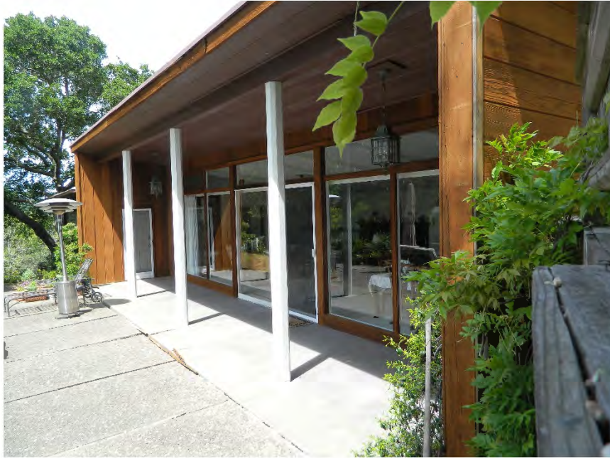
Photo showing the ground floor along the east elevation, facing south.
