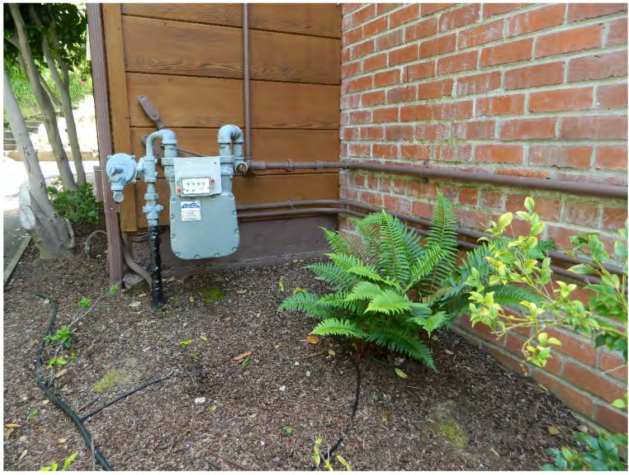
Photo showing the northeast elevation foundation, facing east.
