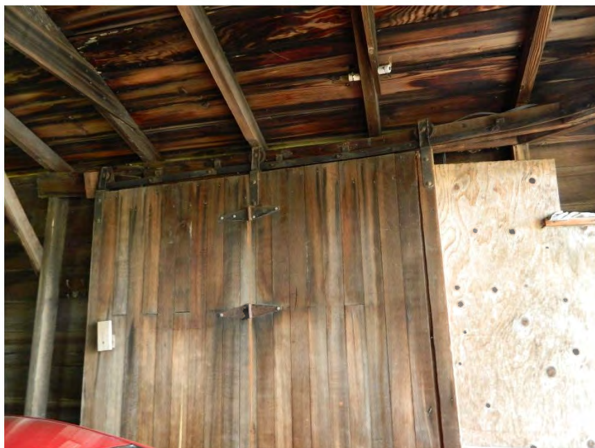
Photo showing the interior of the garage and the original sliding barn-door and track railing.
