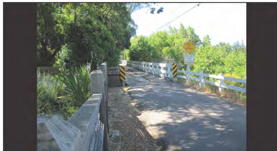
Photo of north end of bridge, facing south.
