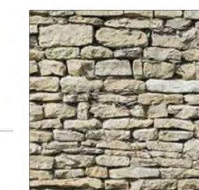
STONE BRICK BASE WALL
