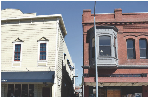
Example of Bay Window and Openings.
