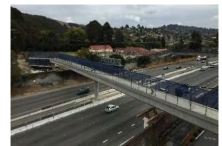
I-80 San Pablo Dam Rd – POC Replacement
