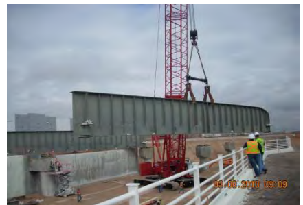
Decatur/UPRR Grade Separation
