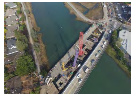
Bon Air Rd Bridge Replacement
