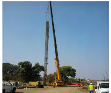
CIDH Bent for Fish Passage at Red Bluff
