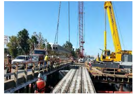
Orwood Rd Bridge Replacement
