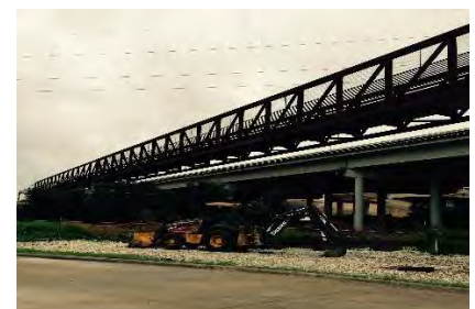
MOPAC – Pedestrian Bridge
