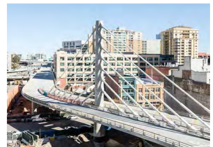
Transbay Bus Ramp Viaduct
