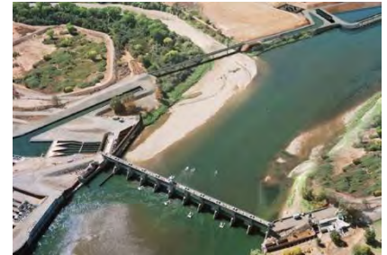
Fish Passage – Red Bluff Diversion Dam
