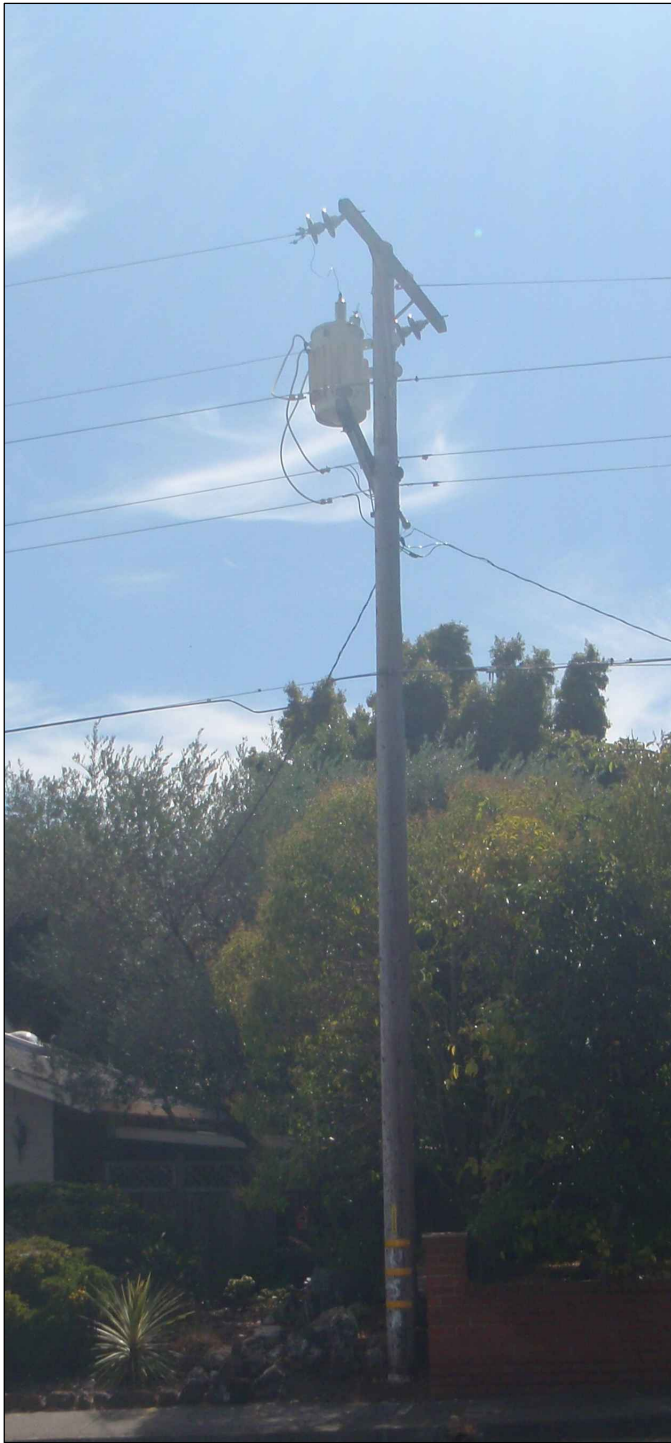
EXISTING POLE PHOTO
