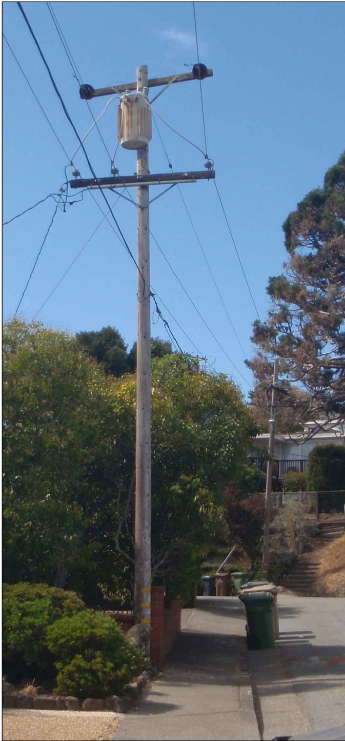
EXISTING POLE PHOTO
