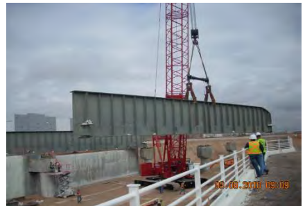
Decatur/UPRR Grade Separation
