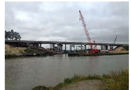
Petaluma River Bridge Replacement
