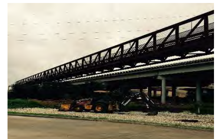
MOPAC – Pedestrian Bridge
