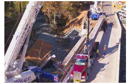
Marsh Creek Rd Bridge Replacement
