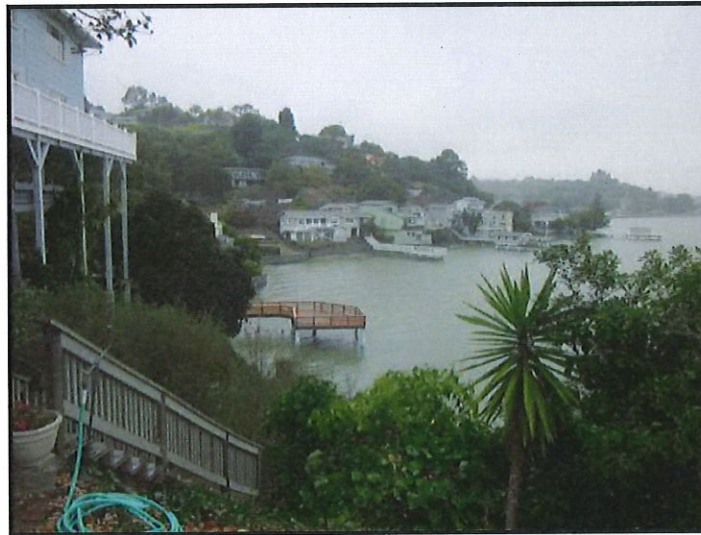
Figure 1: Pt. San Pedro Road beach sewer is under water below the houses visible in the distance.
