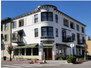
Figure 4.7 Most recent projects have applied for height bonuses and additional height as development concessions.
