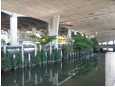
Figure 4.25 Irwin Creek runs underneath US-101 and can be part of a Downtown-wide flood control strategy
