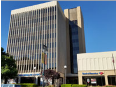
Figure 4.6 Existing building heights in Downtown vary, with a few cases of awkward transitions.
