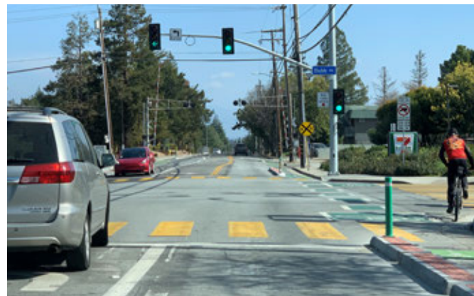
Figure 6.22 Examples of strategies recommended for Downtown's vehicular network: (far left) a high visibility crosswalk with a traffic circle, and (left) a protected left turn and separated bicycle path at a rail crossing.
