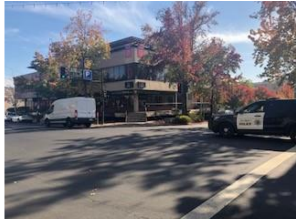
Built project at Fourth and A Streets
