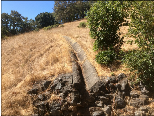
Photo 5 – Concrete lined channel to direct hillside sheet flow during rain events into ephemeral channel. Photo facing south.
