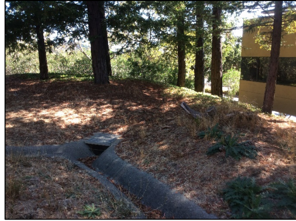
Photo 6 – Concrete drainages to direct hillside sheet flow during rain events into culvert connecting under adjacent development into canal which connects to Gallinas Creek and into San Pablo Bay. Photo facing east.
