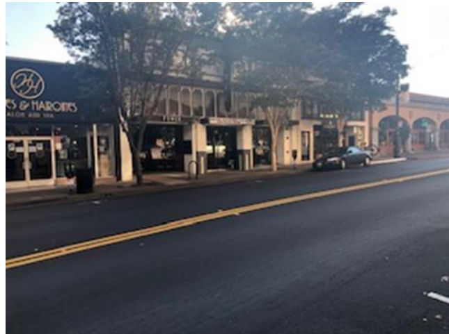
919 Fourth Street with restored transom and glass/upper storefront
