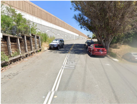
No Bike Lanes No Sidewalks Limited ROW
