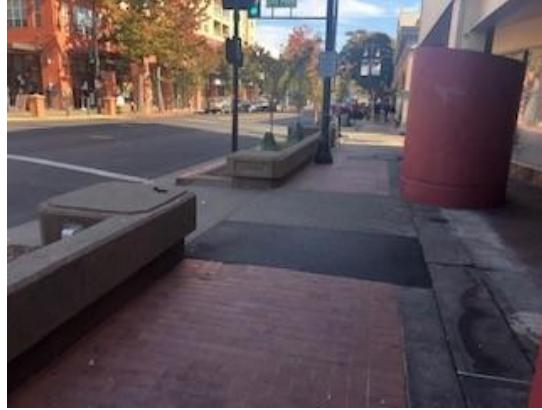
Current, built improvements at Fourth and Court Streets
